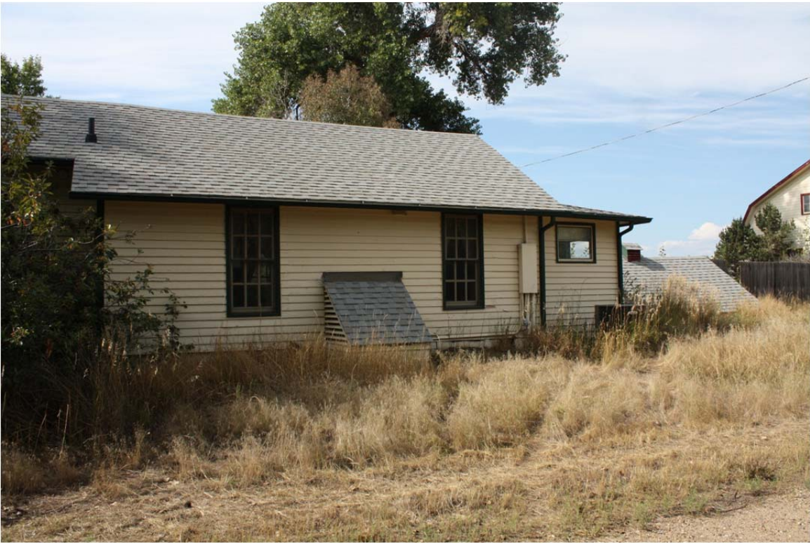
Figure 6. Farmhouse (North Elevation)
