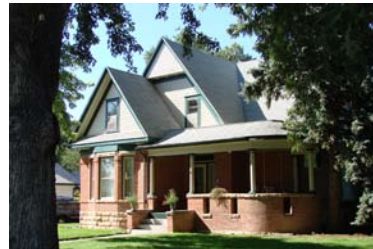
Preserve original brick and stone
