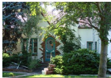
Preserve original stucco
