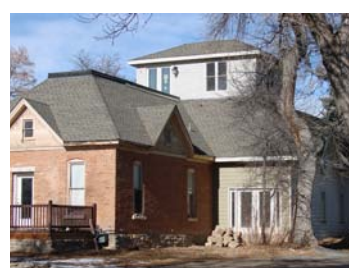
Inappropriate scale and massing of addition
