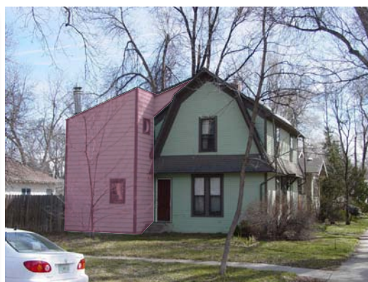
Inappropriate design, massing and roofline of addition
