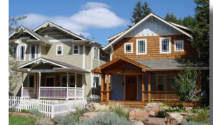
Contemporary materials and colors are appropriate for infill development, provided they are compatible with the character of the historic neighborhood
