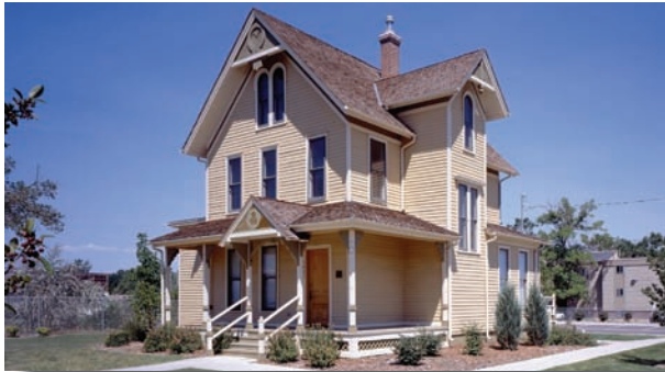
Handicapped access not provided to front porch, so does not adversely impact the primary historic facades
