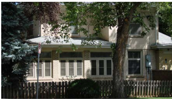
Appropriate porch enclosure using window types that match original house
