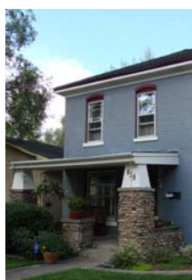
Inappropriate porch architectural style and materials
