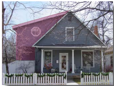
Inappropriate - location and scale of addition
