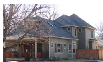
Inappropriate scale and massing of addition
