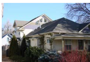
Inappropriate scale and massing of addition
