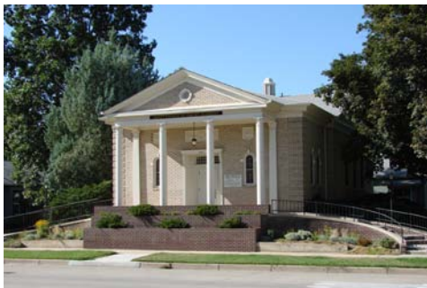
Appropriate location for access provided by ramp up from the side to the main entrance
