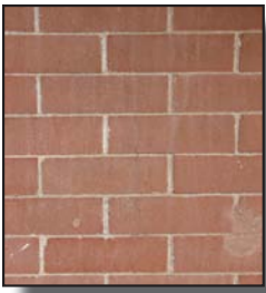
Appropriate cleaning and repointing
