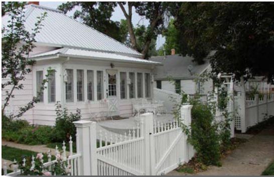
Appropriate fencing design and materials
