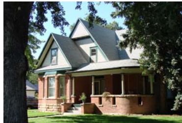
Preserve original brick and stone
