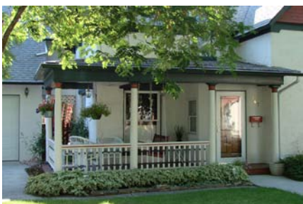
New porch constructed in style compatible with original house
