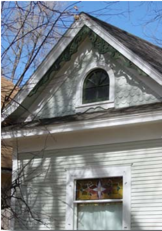
Narrow profile wood bevel lap siding with wood corner trims, wide head trim at fascia and decorative scalloped shingles in gable end
