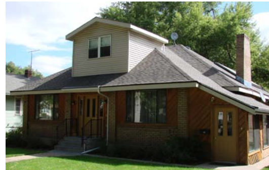
Inappropriate scale and height of dormer
