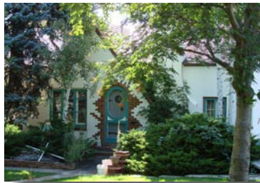
Preserve original stucco
