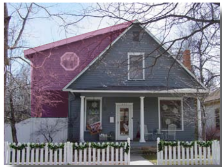
Inappropriate - location and scale of addition
