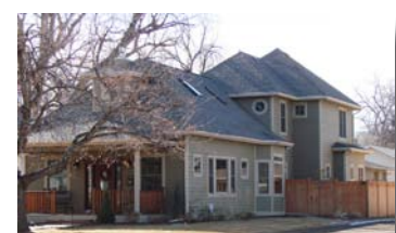
Inappropriate scale and massing of addition
