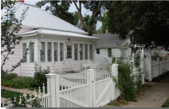
Appropriate fencing design and materials
