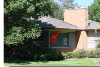
Preserve distinctive corner windows
