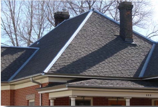
Appropriate replacement fiberglass shingles with metal hip and ridge caps, half-round gutters and round downspouts
