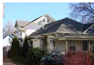
Inappropriate scale and massing of addition
