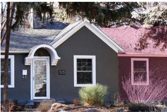
Appropriate scale and roofline of addition, with different stucco texture on the addition
