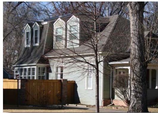
Inappropriate dormer design, massing and roofline
