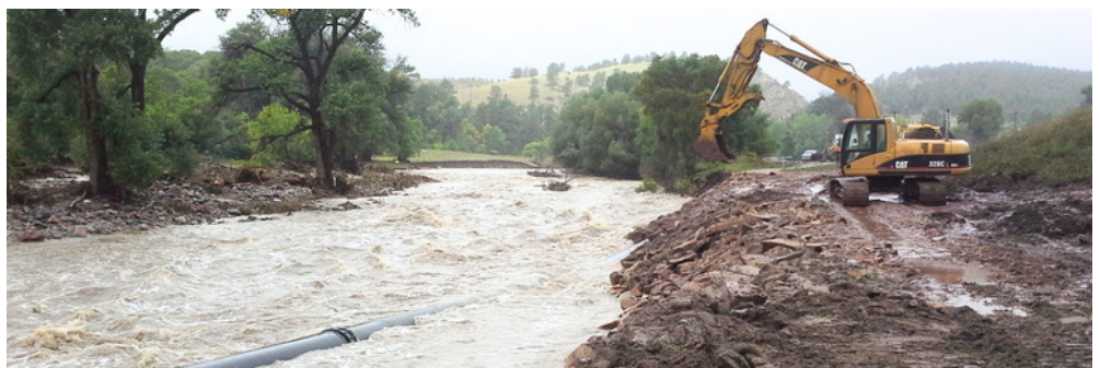
Crews dump rocks from nearby quarry to keep floodwaters from unearthing city water lines.
