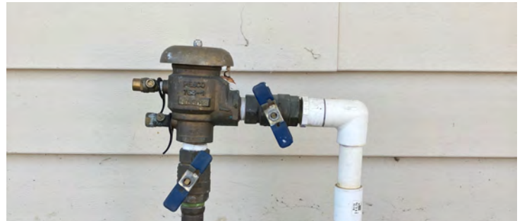
A residential sprinkler system backflow prevention installation
