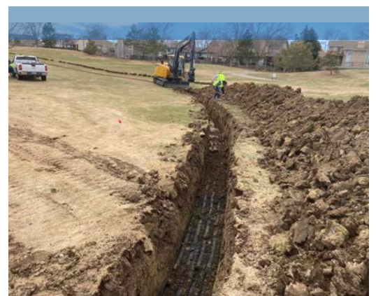
Irrigation Replacement Project at Cattail Creek
