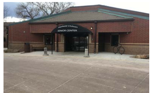
The completed Senior Center entrance ADA project
