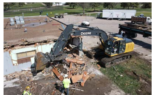
Workers supervise the demo of the old clubhouse
