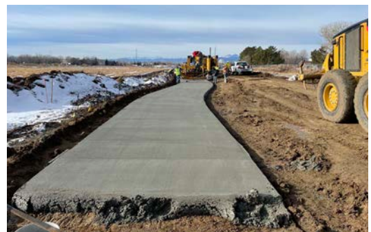
Centerra Trail construction
