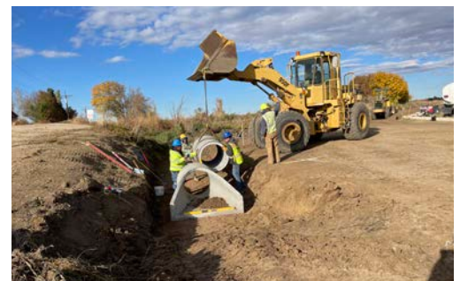
Beginning construction of Centerra Trail
