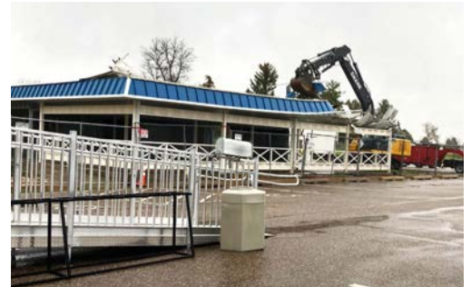
Demo of the old clubhouse begins at The Olde Course
