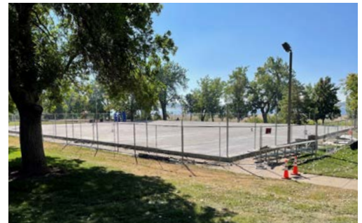
New concrete on North Lake Park basketball courts
