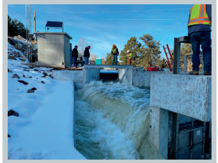
Water from the Loveland Canal rushing through the new GRGRB Diversion Structure. Water hits maximum flow capacity when it reaches 75 cubic feet per second.
