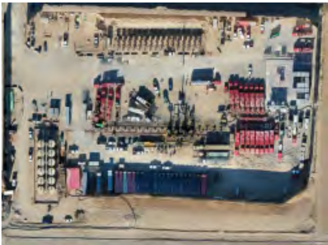
Overhead view of a multiple-well site with hydraulic fracturing equipment set up inside a sound wall
