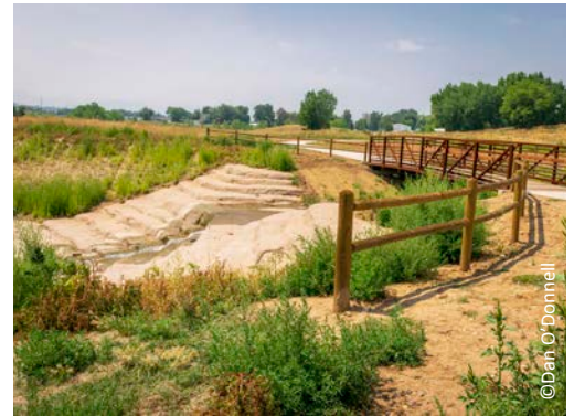
New trail and stormwater outfall at Old St. Louis Natural Area
