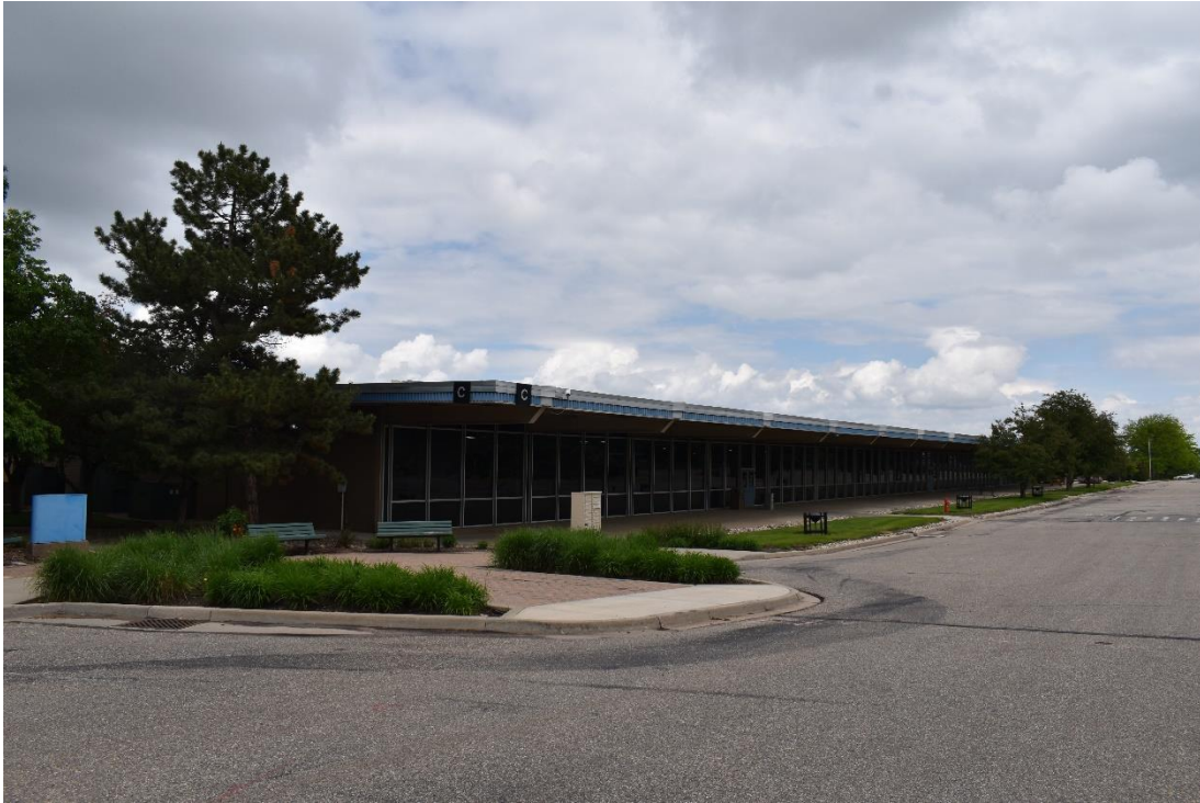
CD 1, Image 25, View to Northeast, of the south wall of Building C
