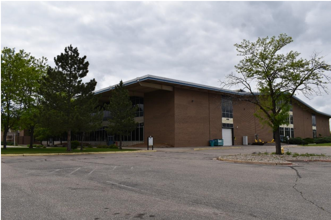
CD 1, Image 44, View to Northwest, primarily of the east wall of Building D
