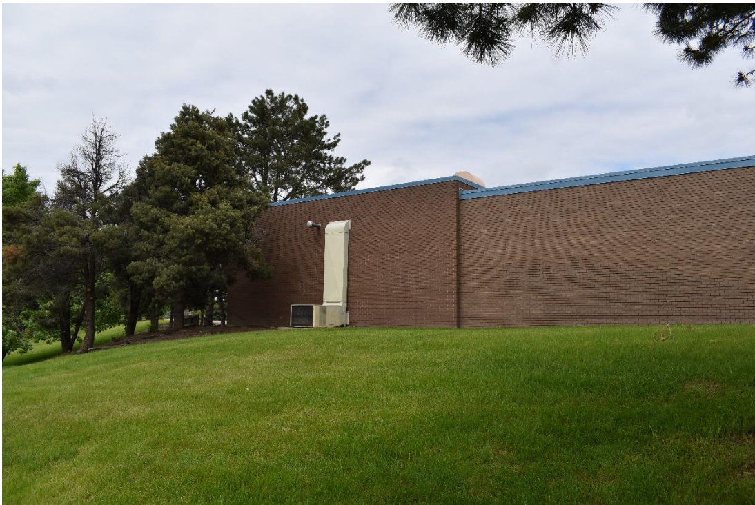
CD 1, Image 56, View to Northeast, of the west wall of the Grounds Maintenance Building
