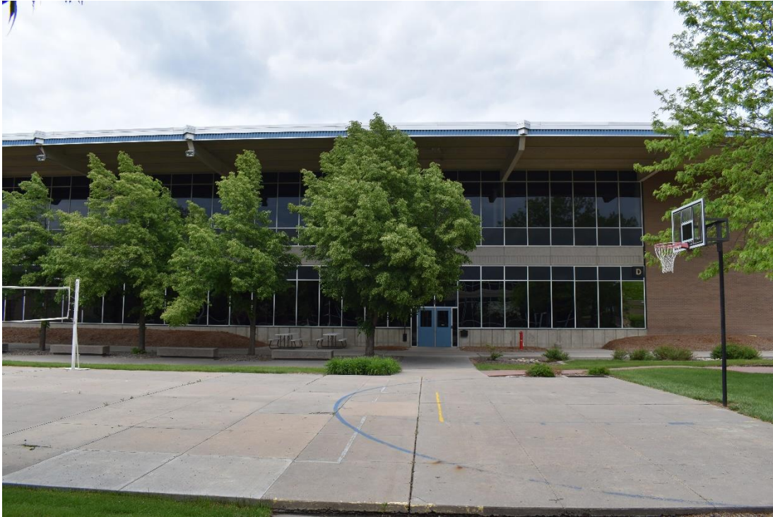
CD 1, Image 45, View to North, of the south wall of Building D
