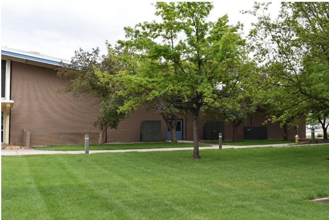
CD 1, Image 24, View to East, of the west wall of Building C
