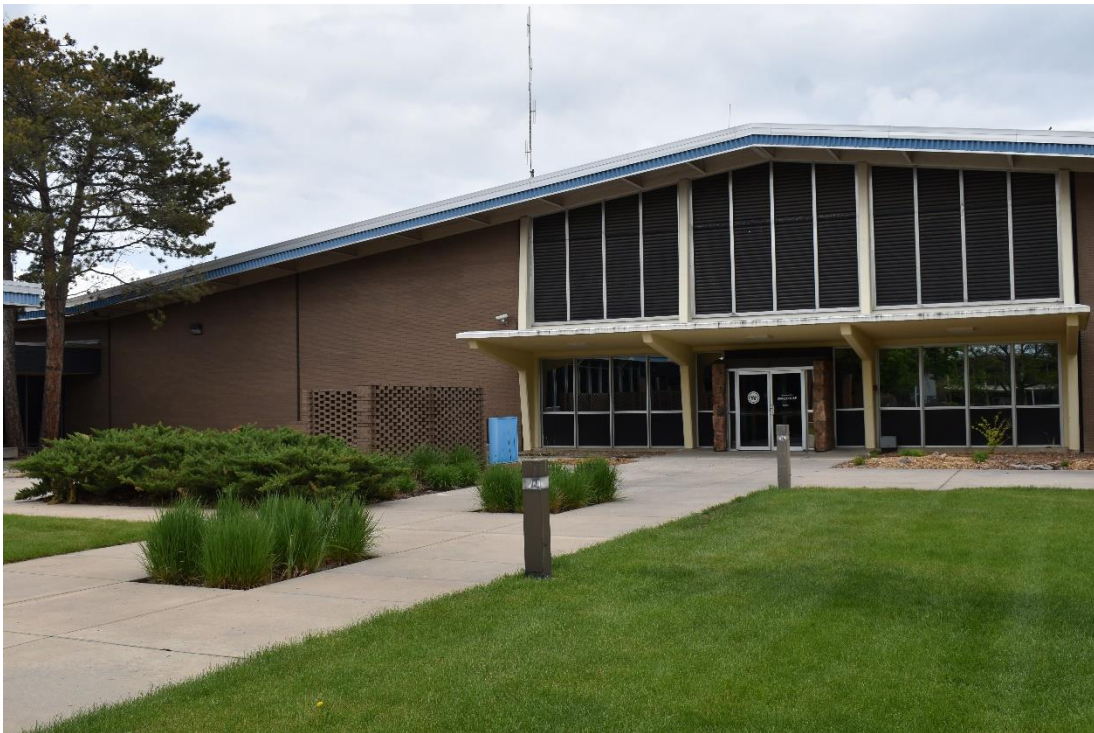
CD 1, Image 22, View to East, of the west wall of Building C
