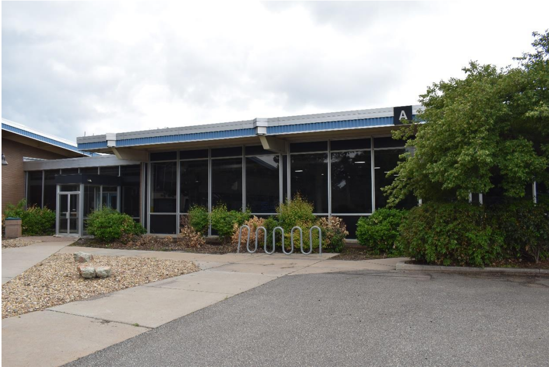
CD 1, Image 11, View to Southeast, of the east end of the north wall of Building A
