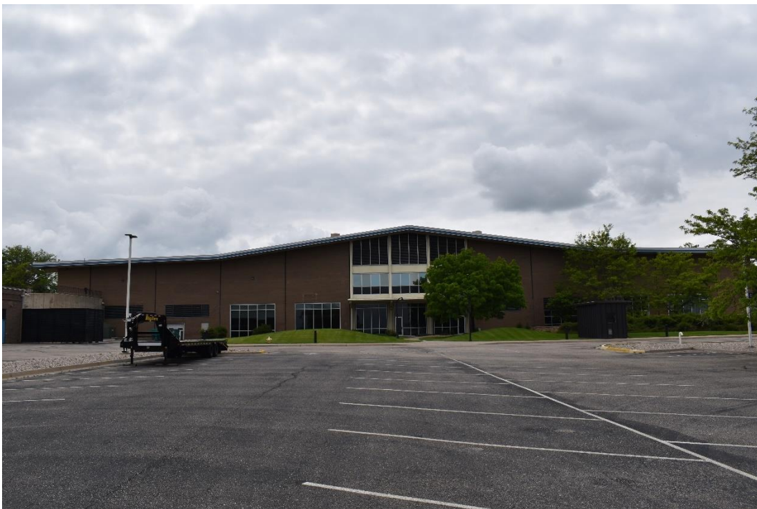
CD 1, Image 28, View to West, of the east wall of Building C
