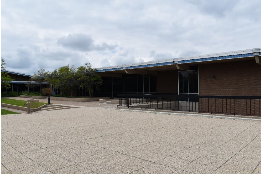
CD 1, Image 47, View to Northwest, of the south wall of Building D
