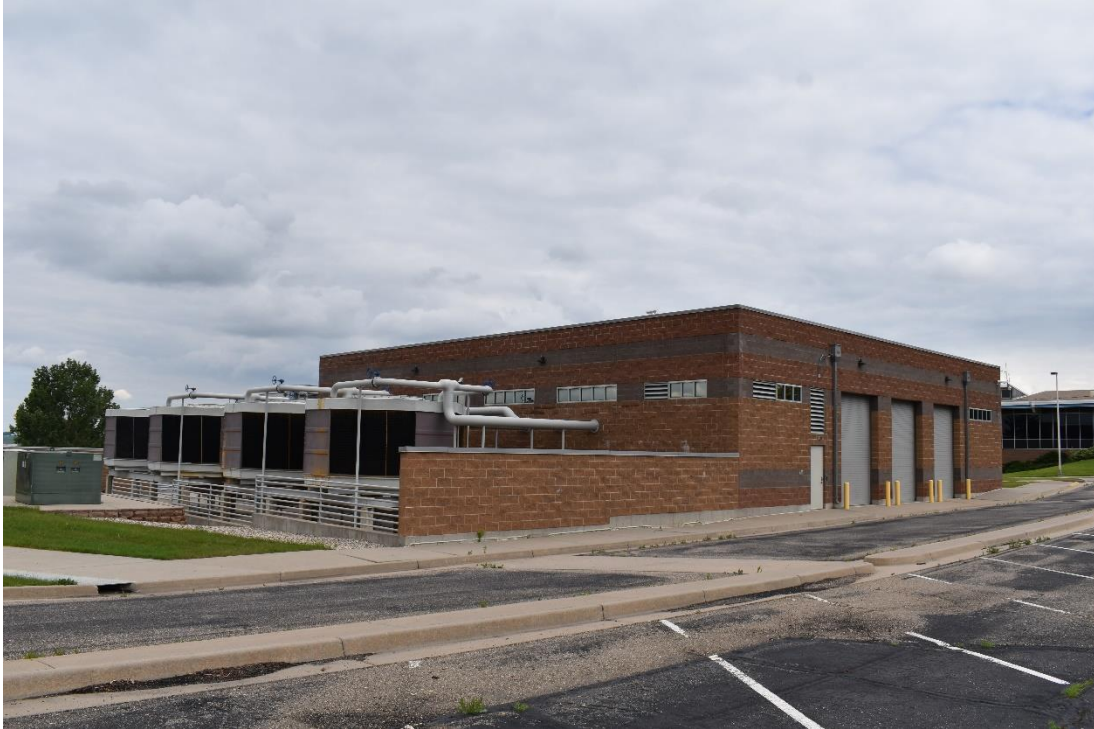
CD 1, Image 52, View to Southeast
