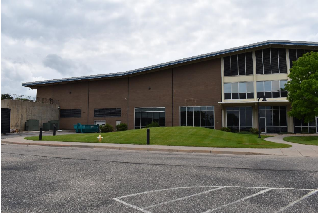
CD 1, Image 29, View to West, of the east wall of Building C
