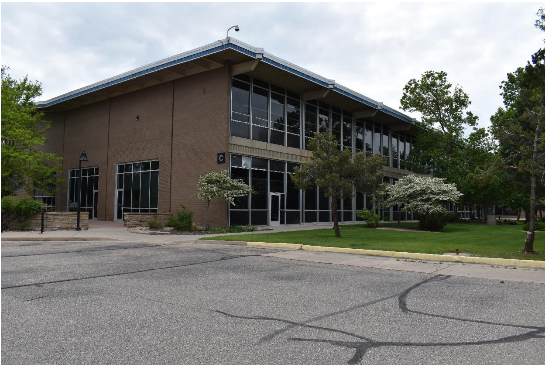
CD 1, Image 32, View to Southwest, of the northeast corner of Building C
