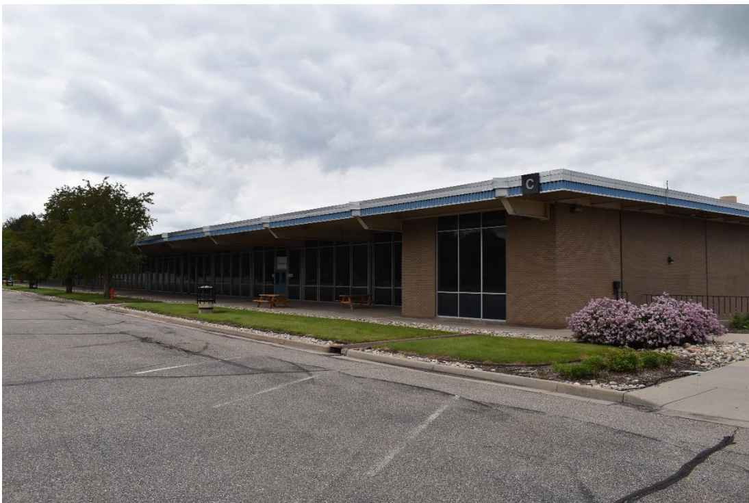
CD 1, Image 26, View to Northwest, of the southeast corner of Building C
