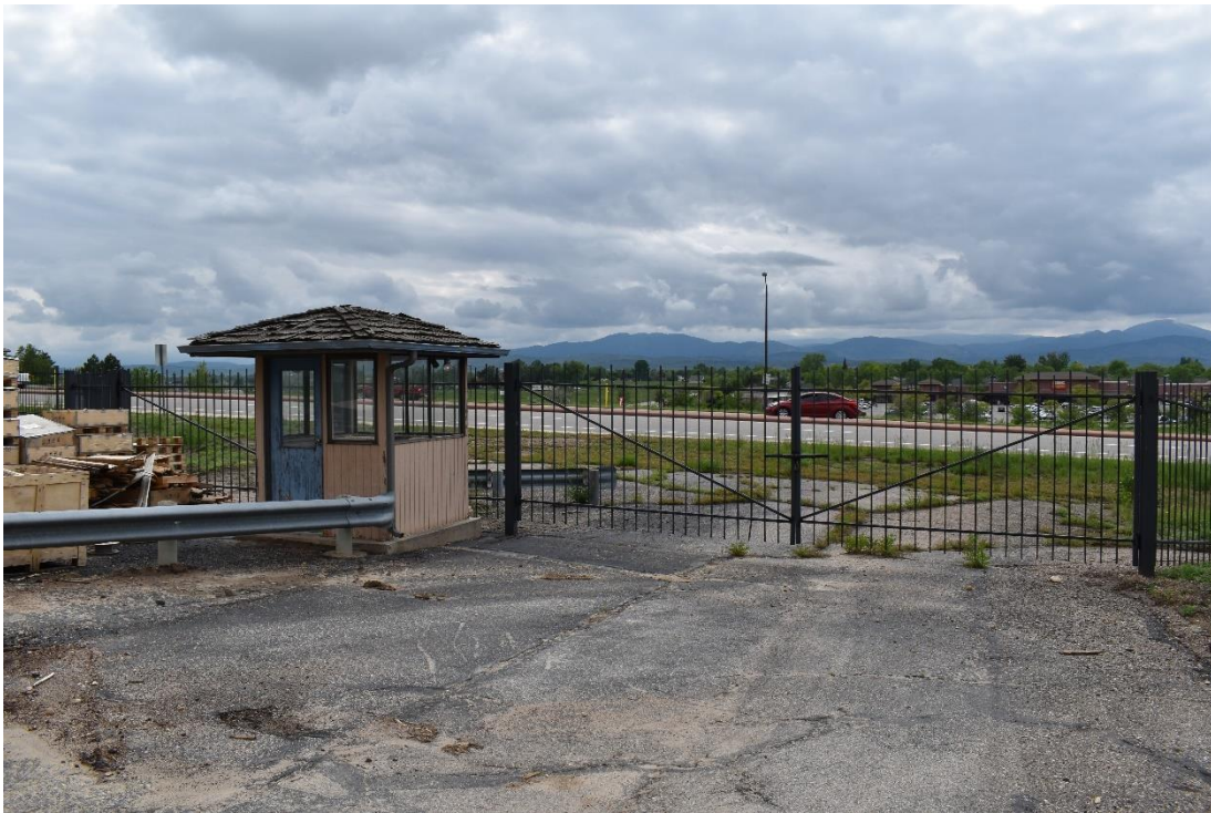
CD 1, Image 58, View to Southwest, of Entrance Station Kiosk and Gate on the west side of the property
