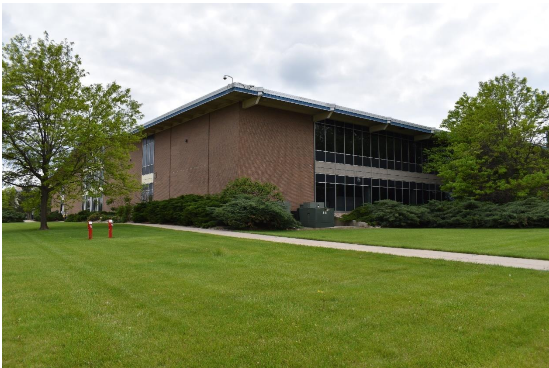
CD 1, Image 42, View to Southwest, of the northeast corner of Building D
