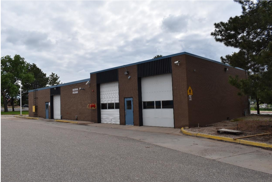
CD 1, Image 53, View to Southwest, of the east and north walls of the Grounds Maintenance Building
