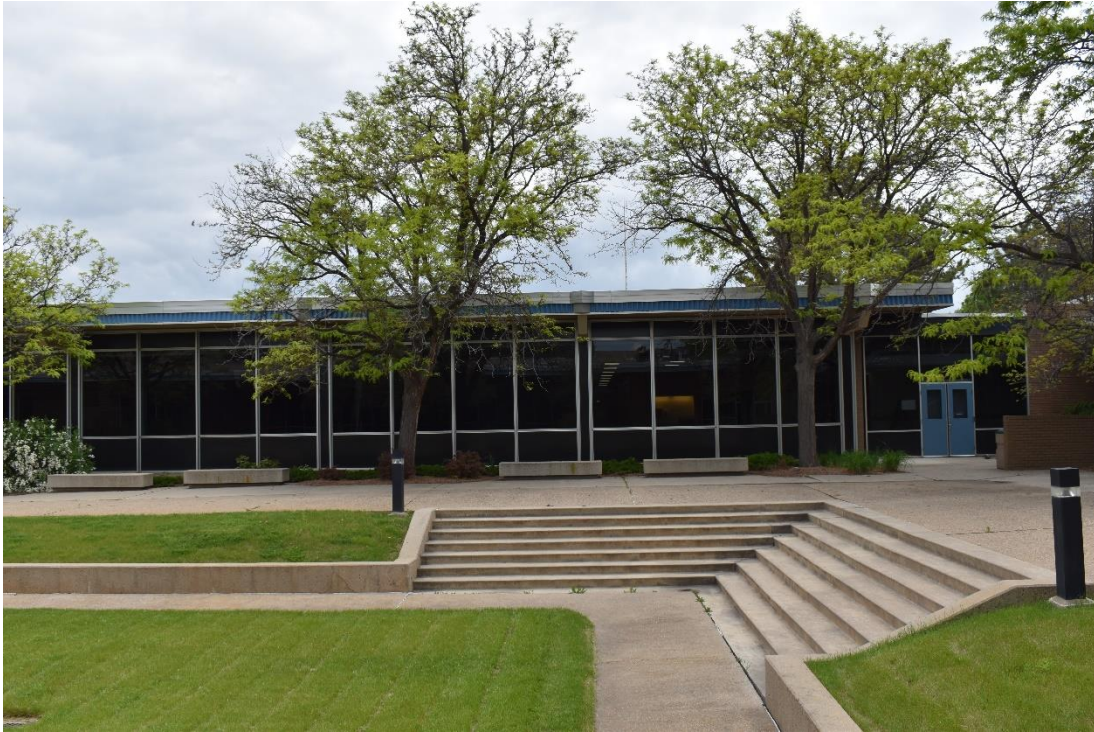
CD 1, Image 33, View to South, of the north wall of Building C
