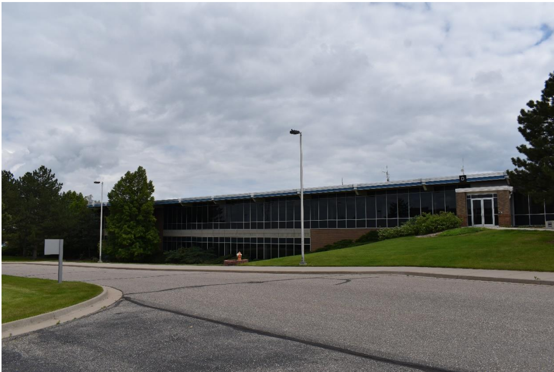
CD 1, Image 38, View to Southeast, of the north wall of Building D
