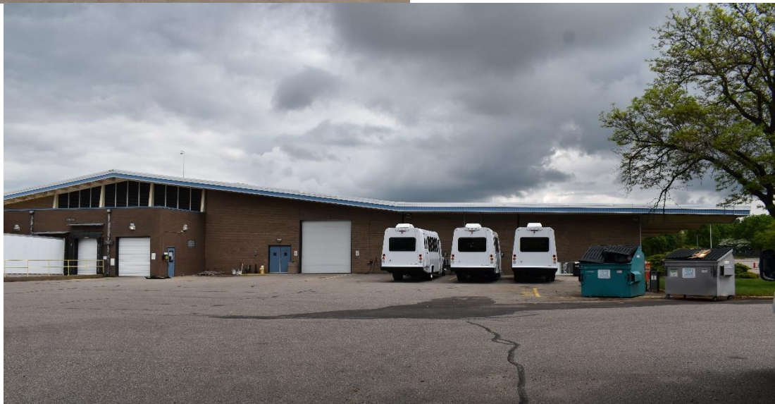
CD 1, Image 6, View to East, of the west wall of Building A
