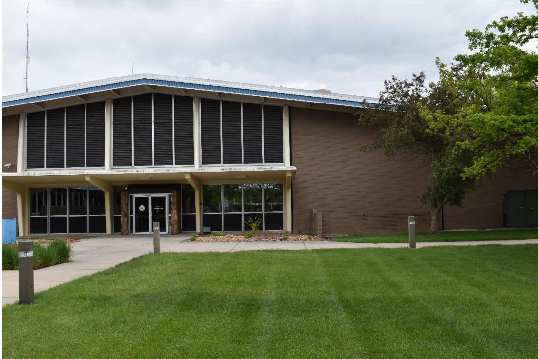
CD 1, Image 23, View to East, of the west wall of Building C
