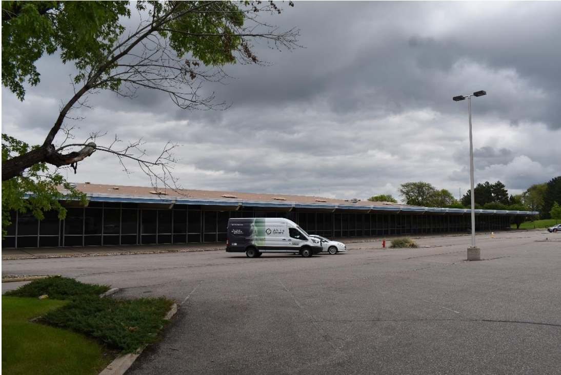
CD 1, Image 1, View to Northeast, of the south wall of Building A
