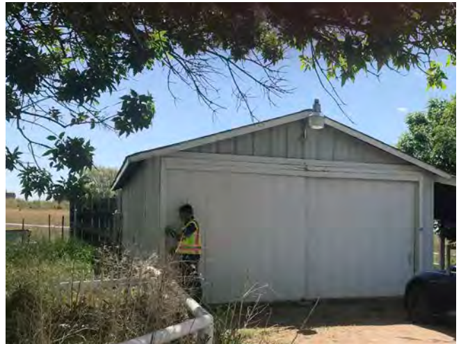
Garage and covered area on the Bonser property
