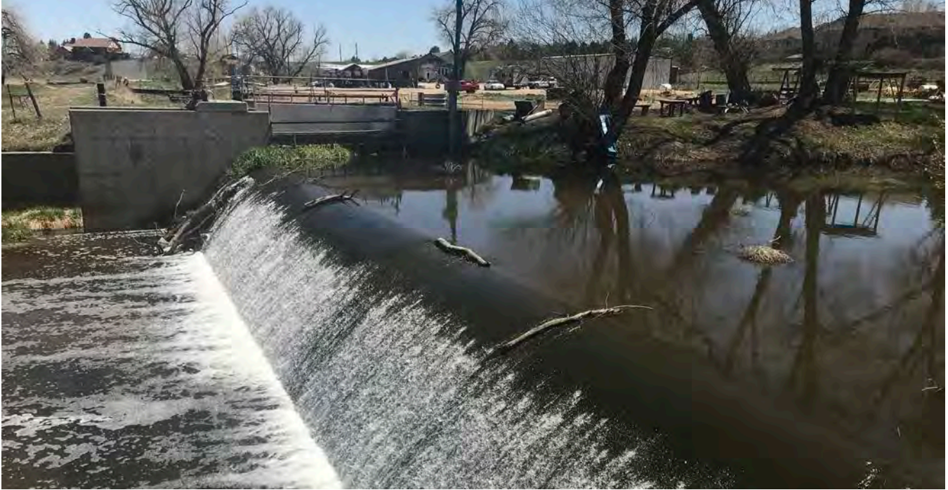
Hillsborough Ditch diversion structure
