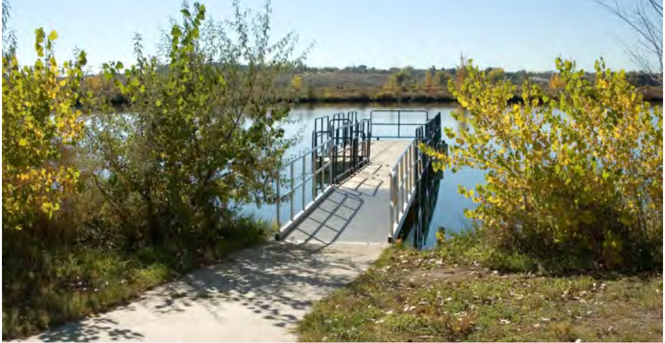
Example of a fishing pier (River's Edge Natural Area)
