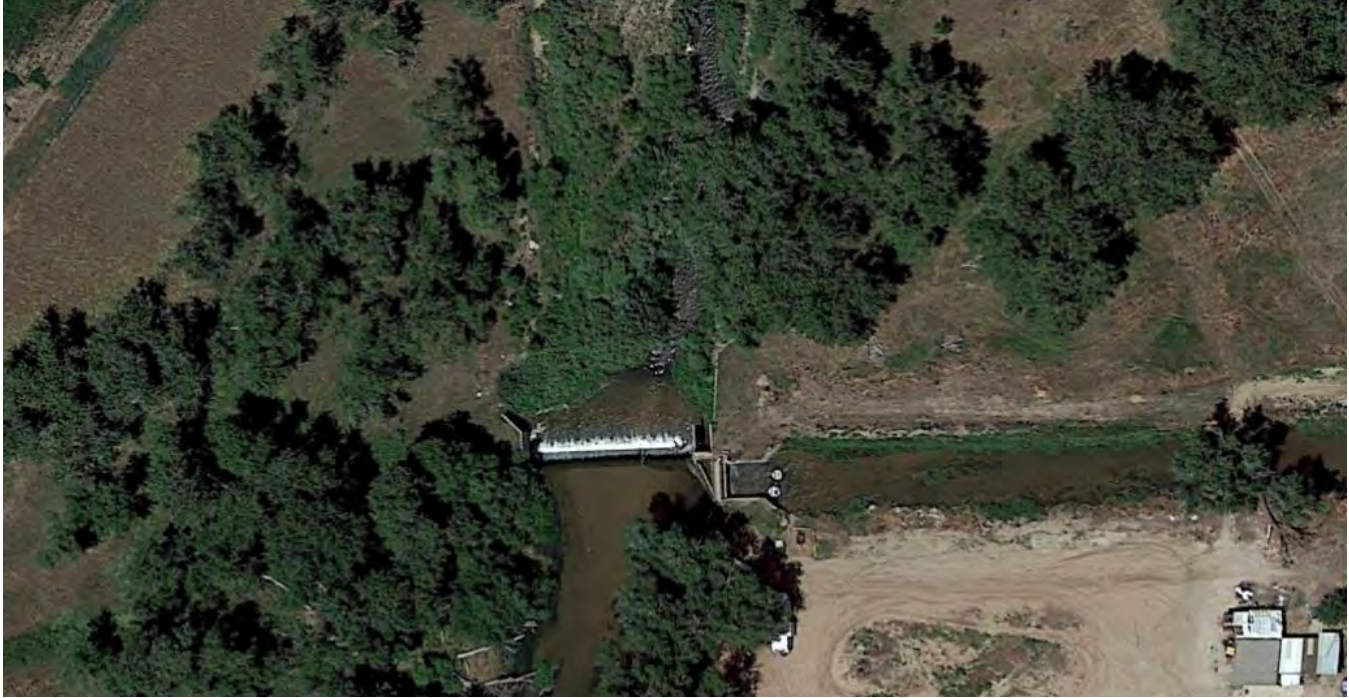
Hillsborough Ditch diversion structure. Google Earth aerial photograph, 2019.
