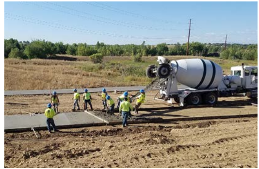
Construction of the Madison Ave. Trail to Old St. Louis
