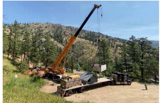
Round Mountain Trail restroom construction
