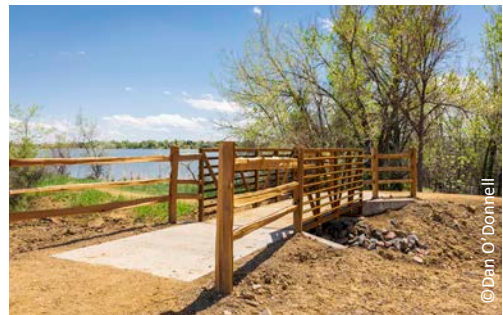
New pedestrian access at Boedecker Bluff
