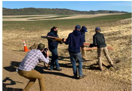
Sign kiosk installation at Prairie Ridge Natural Area
