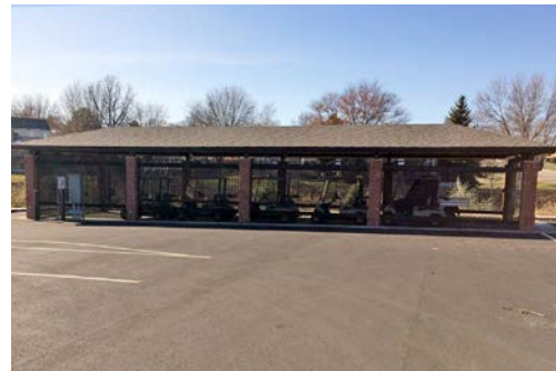
New cart storage building at Cattail Creek
