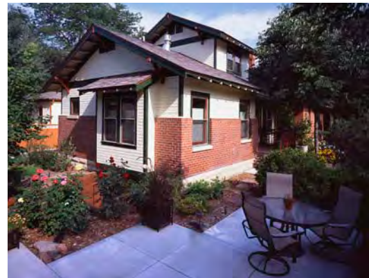
Appropriate scale and articulation of addition
