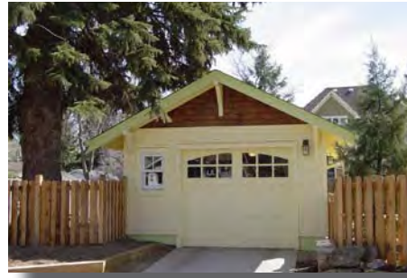
Appropriate detached garage accessed from side street
