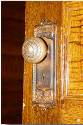
Retain original hardware
