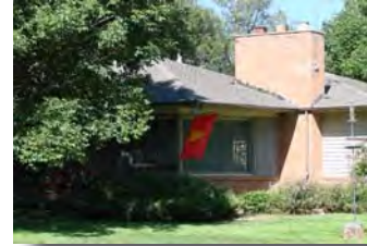
Preserve distinctive corner windows
