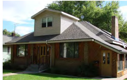
Inappropriate scale and height of dormer
