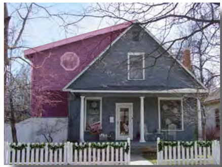
Inappropriate - location and scale of addition
