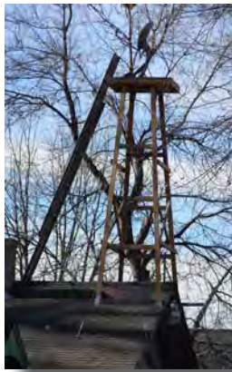
Inappropriate satellite dish installation
