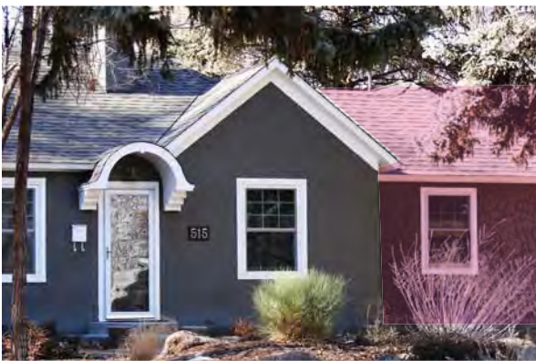
Appropriate scale and roofline of addition, with different stucco texture on the addition
