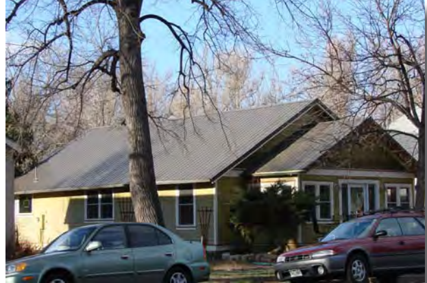
Reroofing original houses with metal roofing is discouraged
