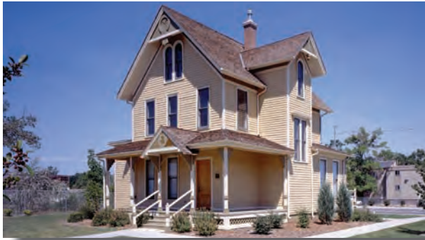
Handicapped access not provided to front porch, so does not adversely impact the primary historic facades
