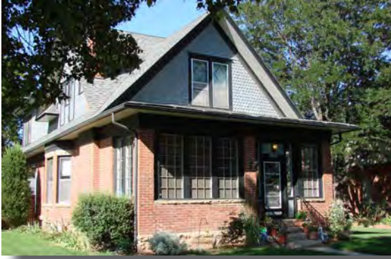
Appropriate porch enclosure maintaining original structural brick columns
