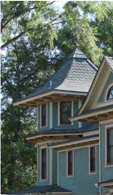
Windows in additions should be compatible with the originals in type, sizes, design and detailing
