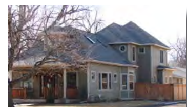
Inappropriate scale and massing of addition
