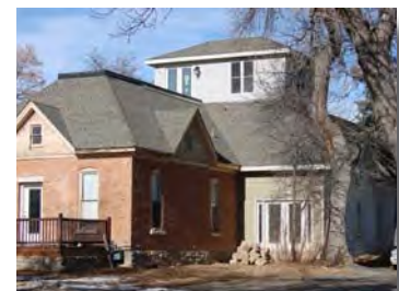
Inappropriate scale and massing of addition
