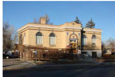
Inappropriate access that adversely impacts the historic character of the building's primary facade
