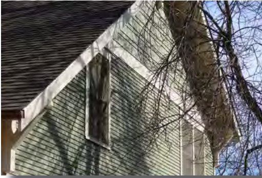
Narrow profile wood bevel lap siding with alternating bands of butt wood shingles in gable end
