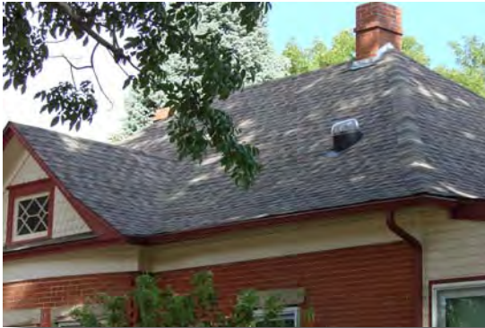
Appropriate solar "tube" installation
