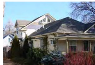
Inappropriate scale and massing of addition
