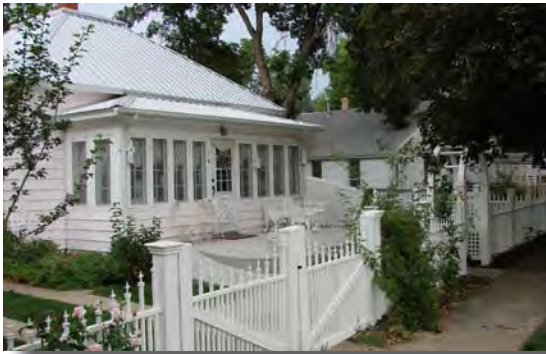
Appropriate fencing design and materials
