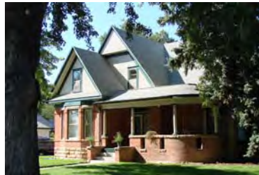
Preserve original brick and stone
