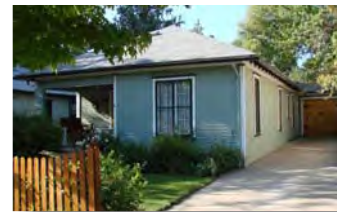
Original wood storm windows preserved
