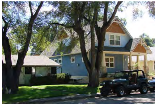
New development that is out of scale to adjacent existing houses
