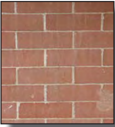
Appropriate cleaning and repointing
