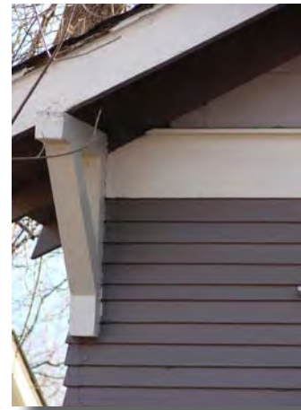
Narrow profile wood bevel lap siding with pre-formed metal corners
