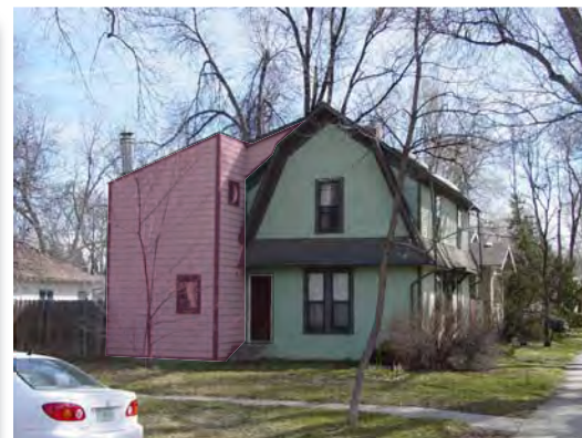
Inappropriate design, massing and roofline of addition
