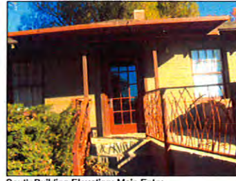
South Building Elevation: Main Entry
