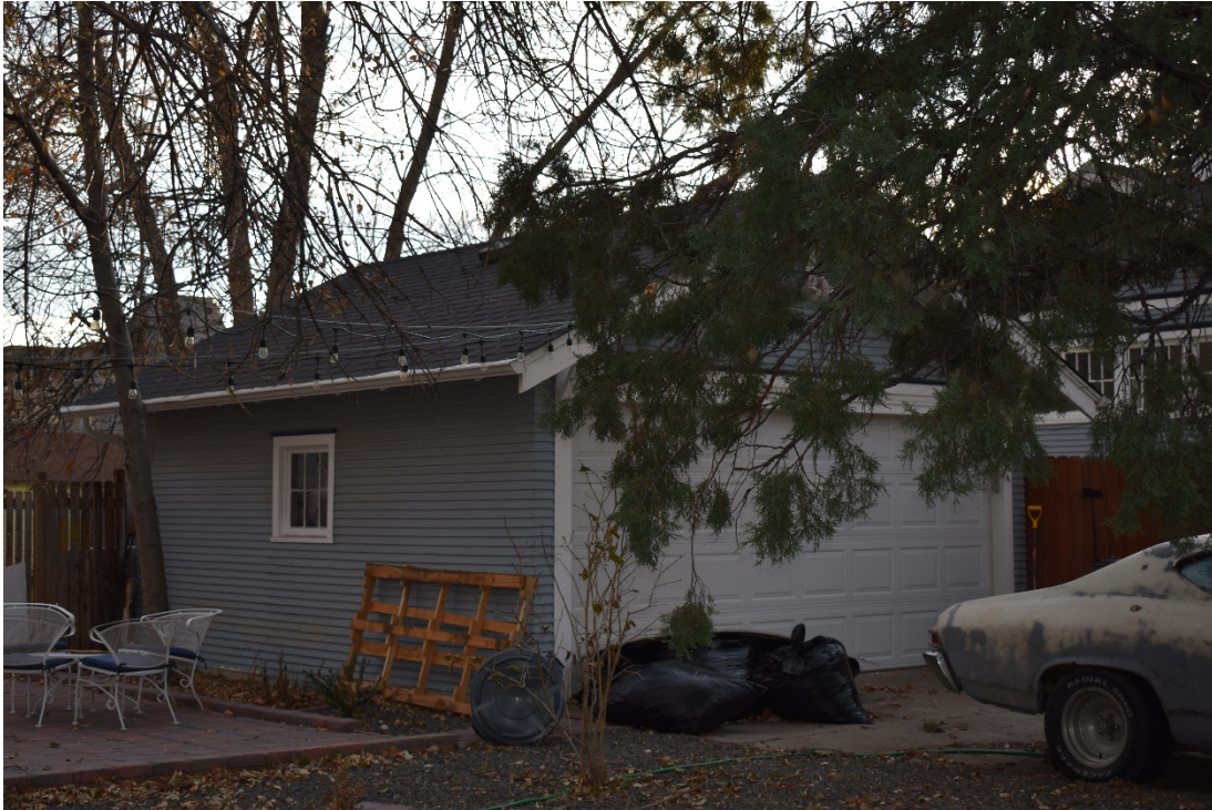
CD 1, Image 165, View to Southwest, of the garage
