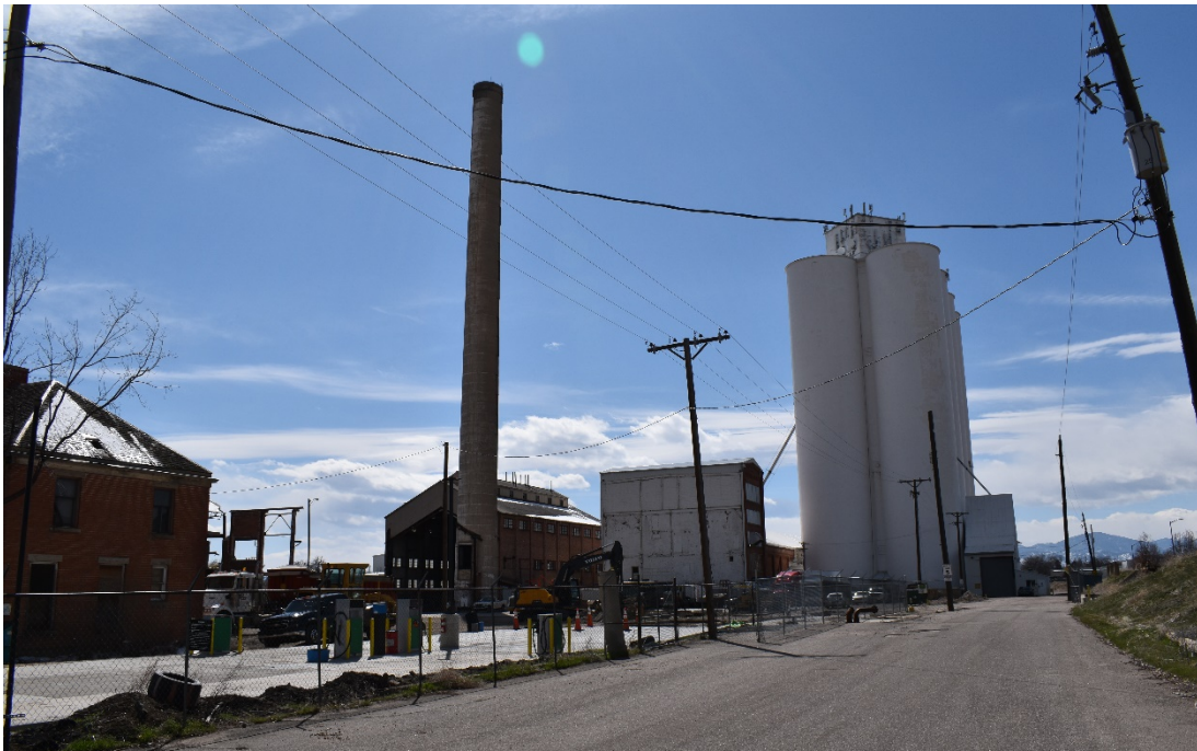
CD 2, Image 10, View to West of the north end of the main office building, the smokestack, partially demolished brick buildings, and the concrete silos assemblage. Photo taken from access road below 11 th Street along the property's northern boundary.
