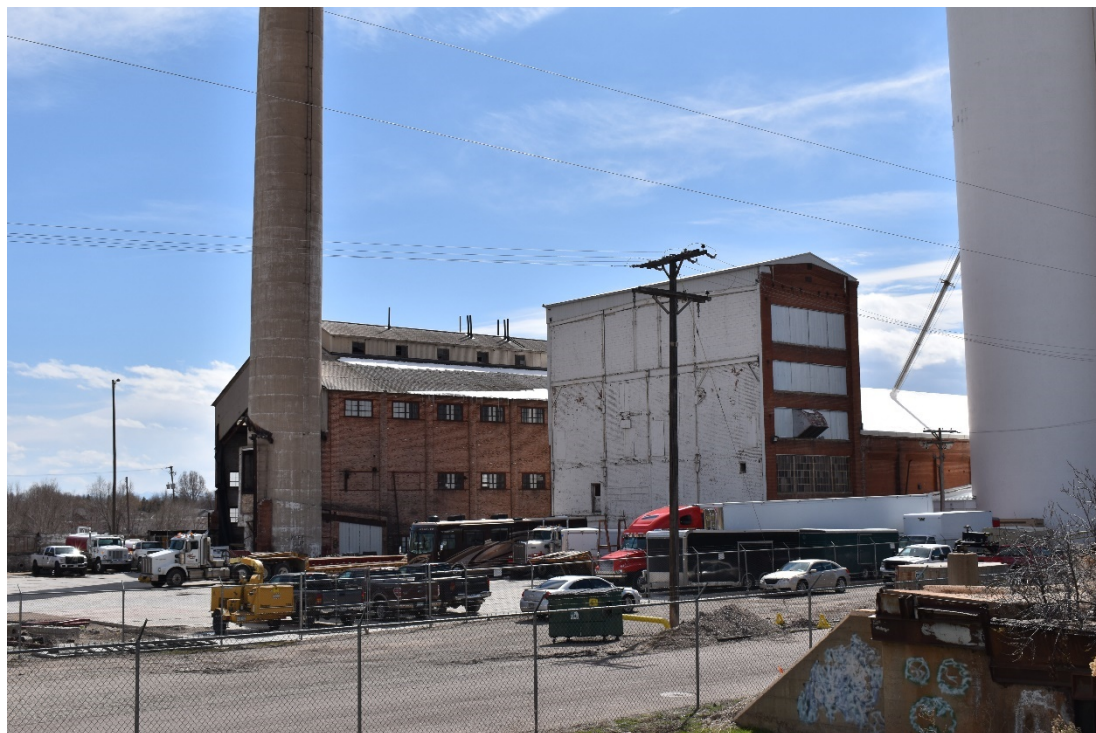
CD 2, Image 2, View to Southwest of brick buildings and lower section of smokestack. Photo taken from 11 th Street.
