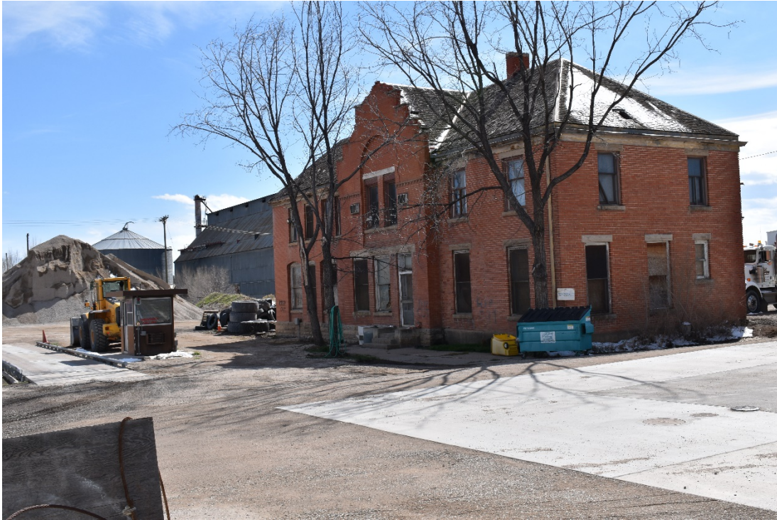
CD 2, Image 11, View to Southwest of the north and east sides of the main office building. The main gable-roofed section to the south was built in 1901. The hipped-roof section at the north end was erected between 1918 and 1927. Photo taken from near 11 th Street.
