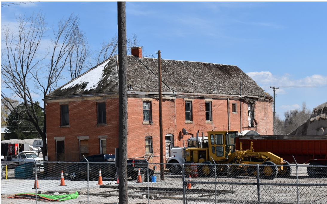
CD 2, Image 6, View to Southeast, of the north and west sides of the main office building. The main gable-roofed section to the south was built in 1901. The hipped-roof section at the north end was erected between 1918 and 1927. Photo taken from 11 th Street.
