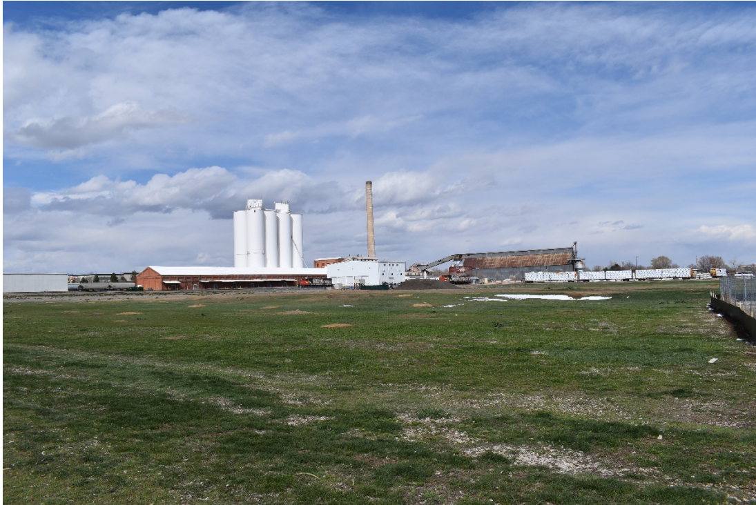
CD 2, Image 23, View to Northeast. Photo taken from near Hayes Avenue.
