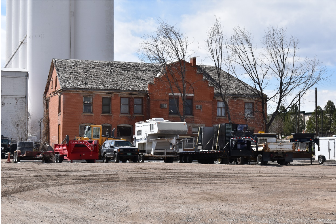
CD 2, Image 13, View to West-northwest, of the east and south sides of the main office building. The main gable-roofed section to the south was built in 1901. The hipped-roof section at the north end was erected between 1918 and 1927. Photo taken from Madison Avenue.
