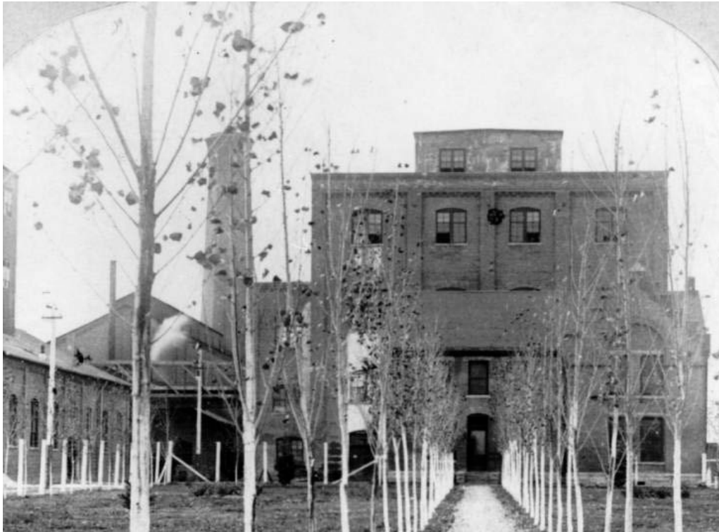
Loveland Great Western Sugar Factory, 1902. View to west, of the east façade of the main office / chemical laboratory building, with the main factory building behind. Photo courtesy of Denver Public Library Digital Collections, call no. x-12199.
