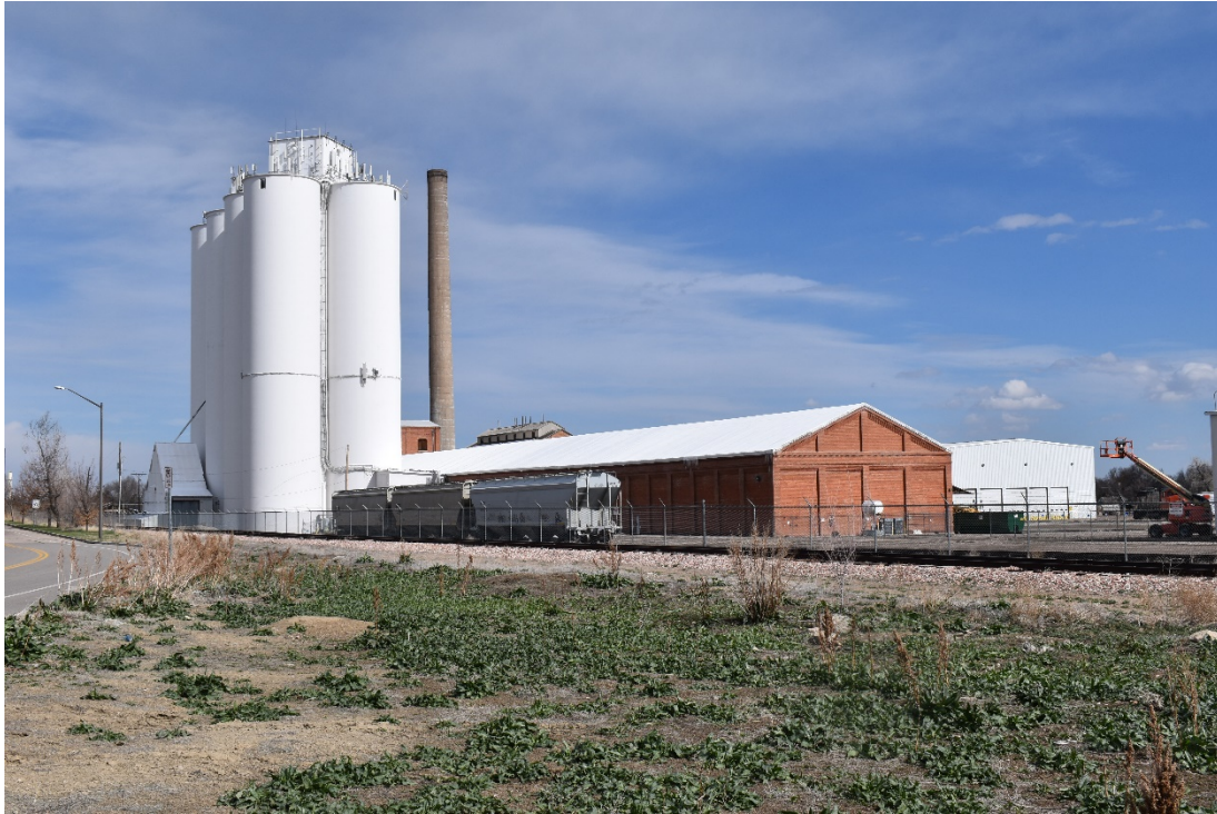
CD 2, Image 27, View to Southeast of a brick building, the concrete silos assemblage, and the smokestack. Photo taken from near the intersection of 11 th Street and Redwood Drive.
