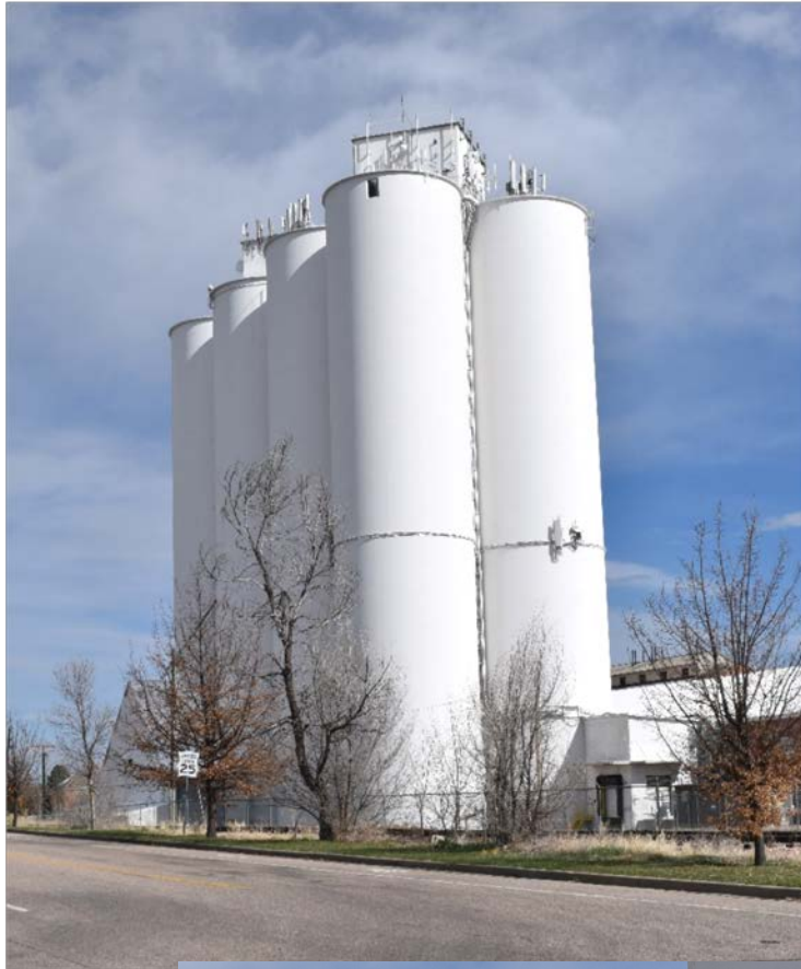
CD 2, Image 29, View to Southeast of the concrete silos assemblage. Photo taken from 11 th
