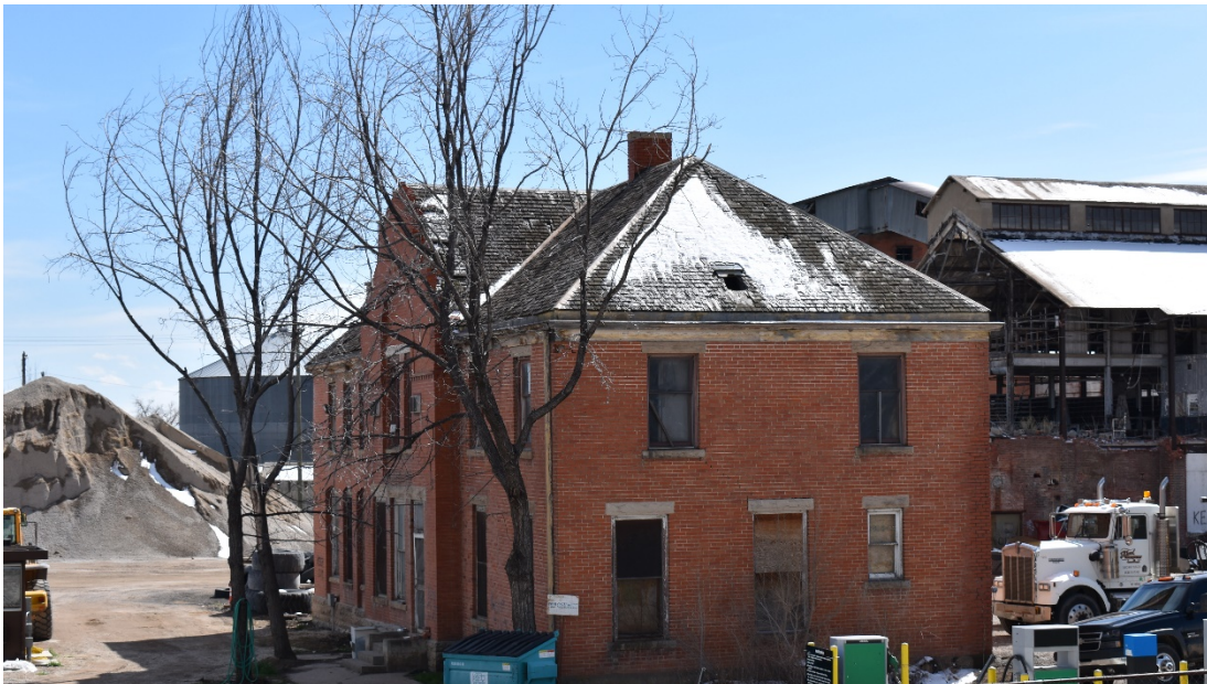
CD 2, Image 8, View to South-southwest of the north and east sides of the main office building. The main gable-roofed section to the south was built in 1901. The hipped-roof section at the north end was erected between 1918 and 1927. Photo taken from near 11 th Street.
