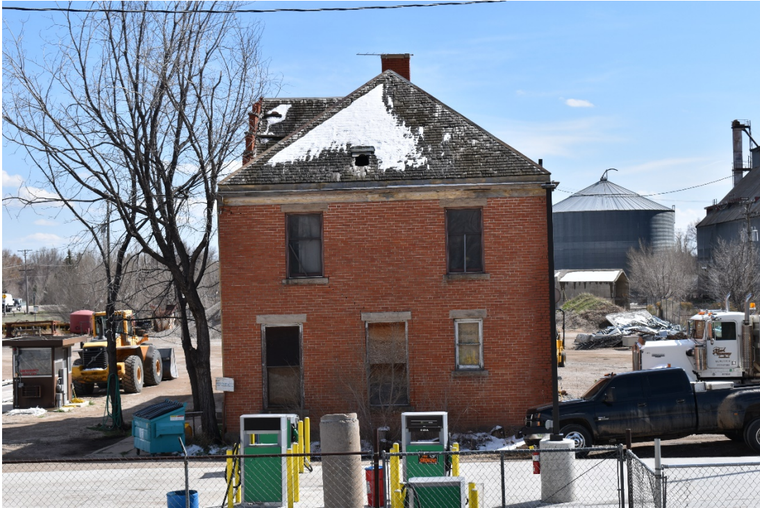
CD 2, Image 7, View to South of the west end of the main office building. The main office building was erected in 1901. The hipped-roof west end, depicted here, is an addition to the original building, erected between 1918 and 1927.
