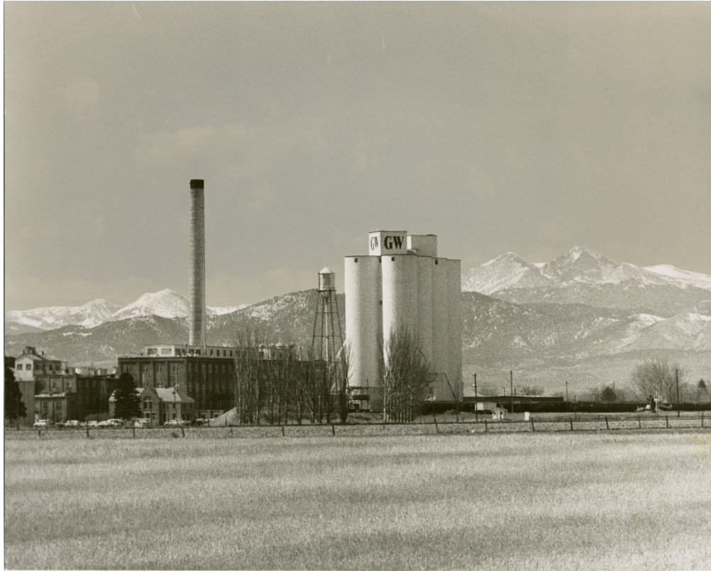
Loveland Great Western Sugar Factory, 1965. View to southwest, with Longs Peak and Mt. Meeker in the right background. Photo courtesy of the Records of the Great Western Sugar Company Agricultural and Natural Resources Archives, Colorado State University, file #AGWS0323.jpg.
