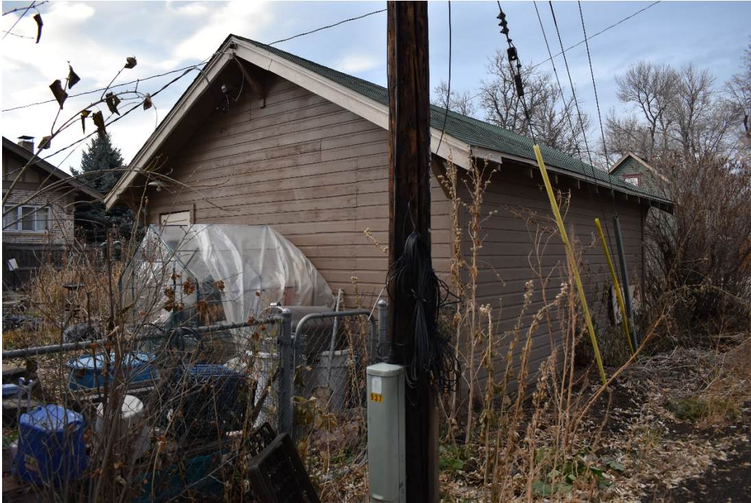
CD 1, Image 172, View to Northwest, of the garage
