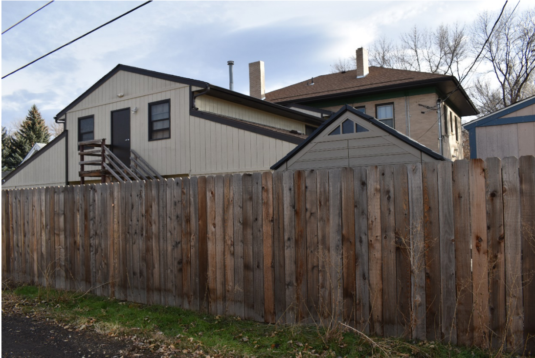
CD 1, Image 135, View to Southeast
