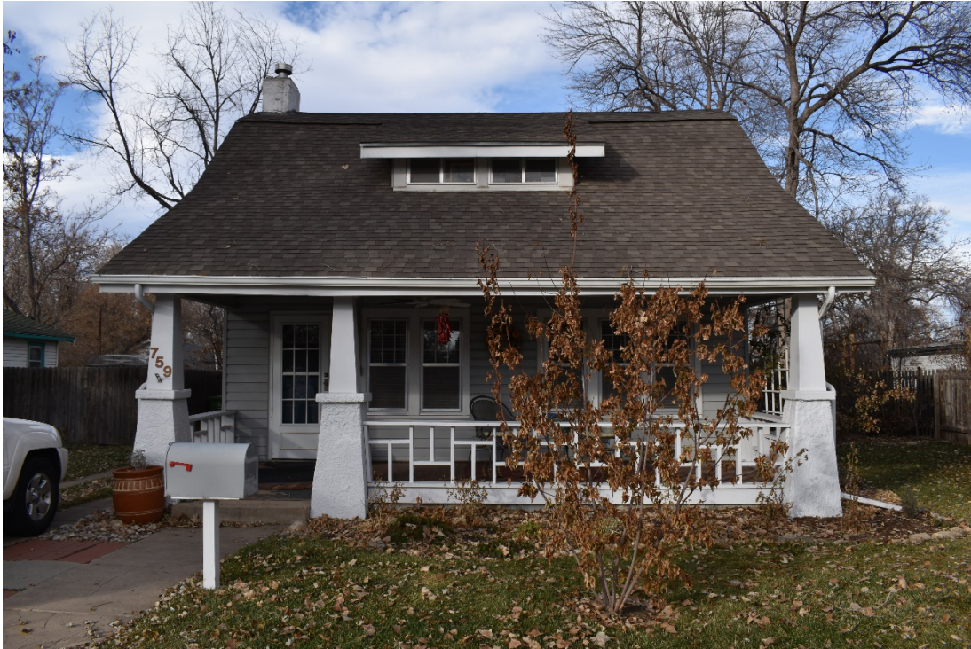
CD 1, Image 123, View to North, of the dwelling
