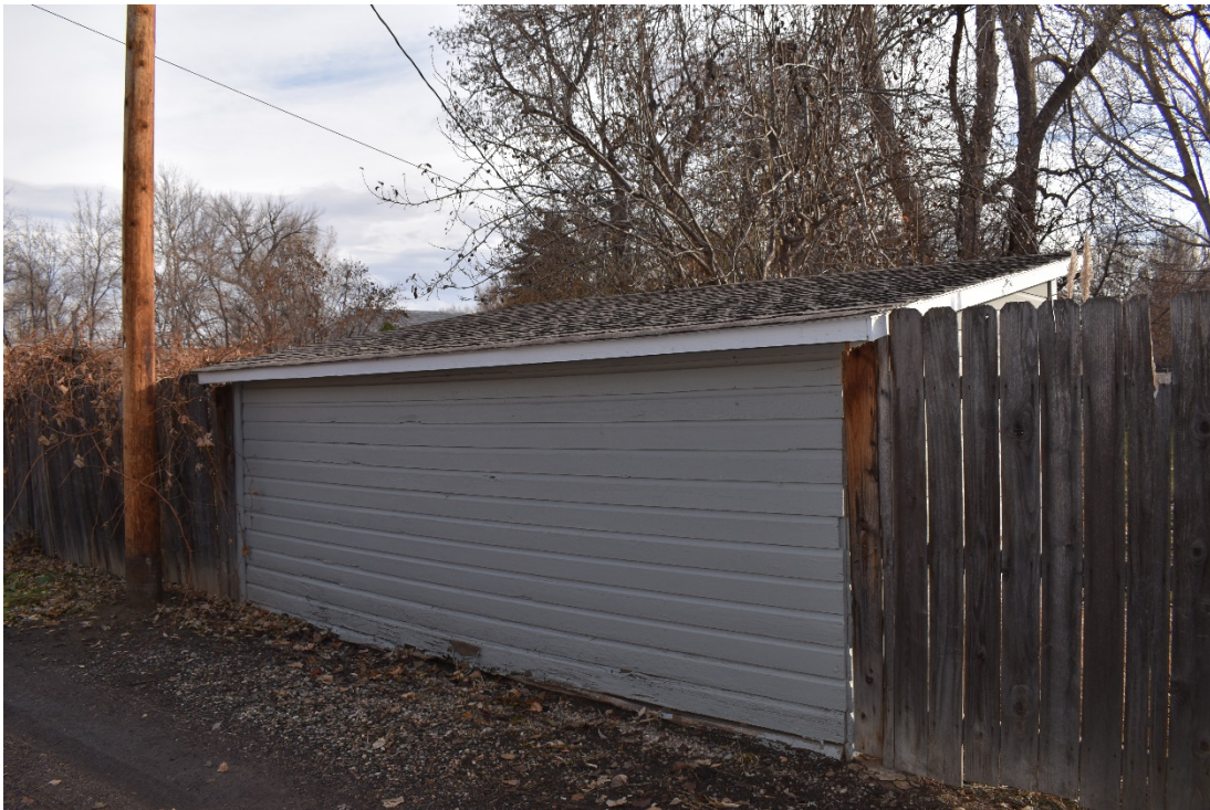
CD 1, Image 130, View to Southeast, of the shed
