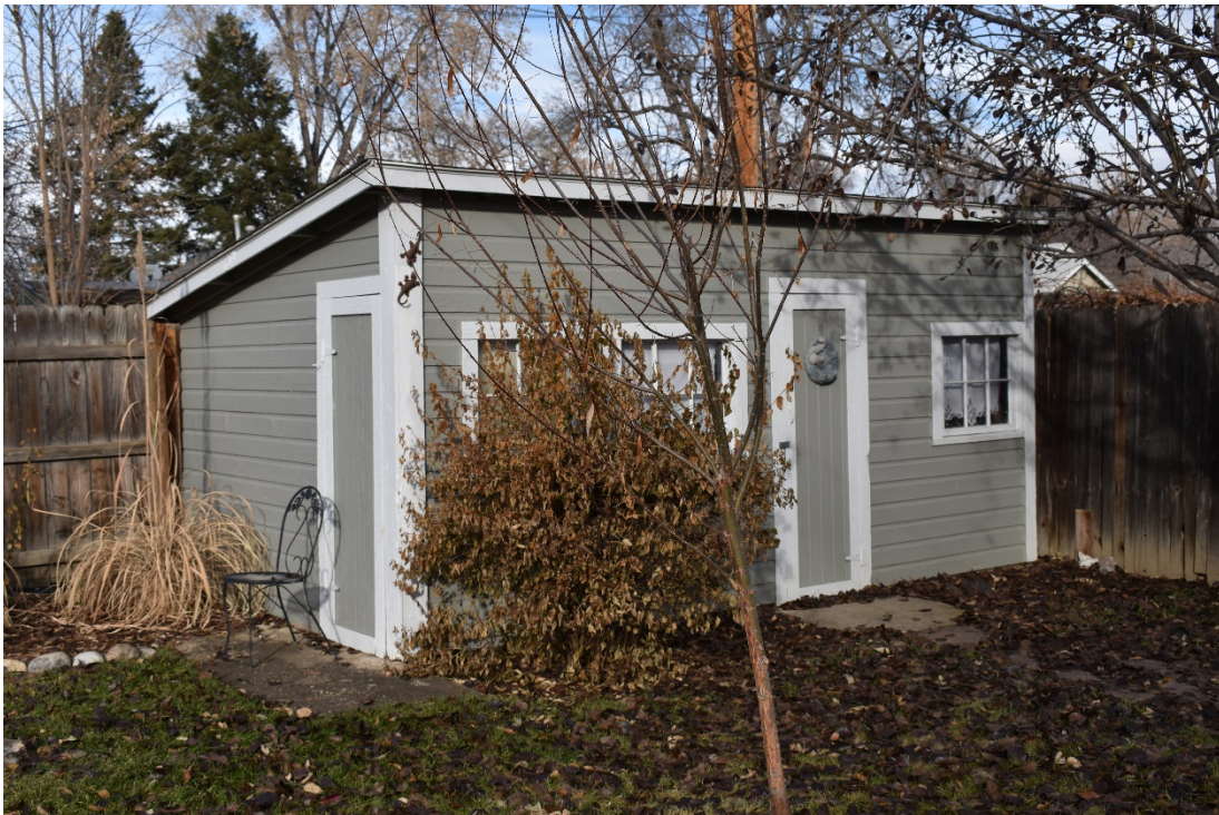
CD 1, Image 128, View to Northeast, of the shed
