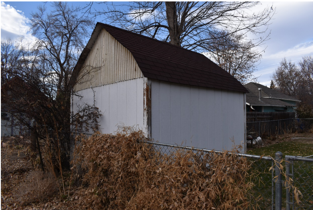
CD 1, Image 122, View to Northwest, of the shed
