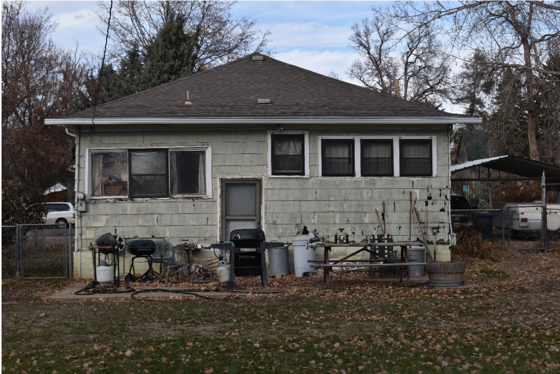
CD 1, Image 121, View to North, of the dwelling
