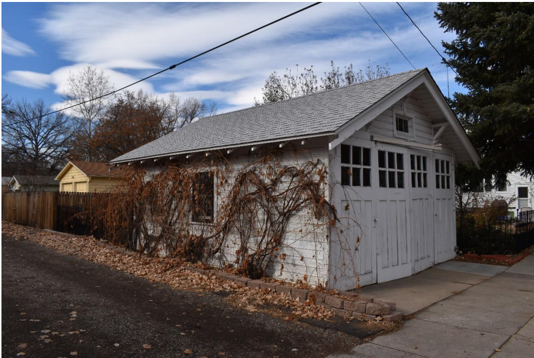
CD 1, Image 108, View to Northwest, of the garage
