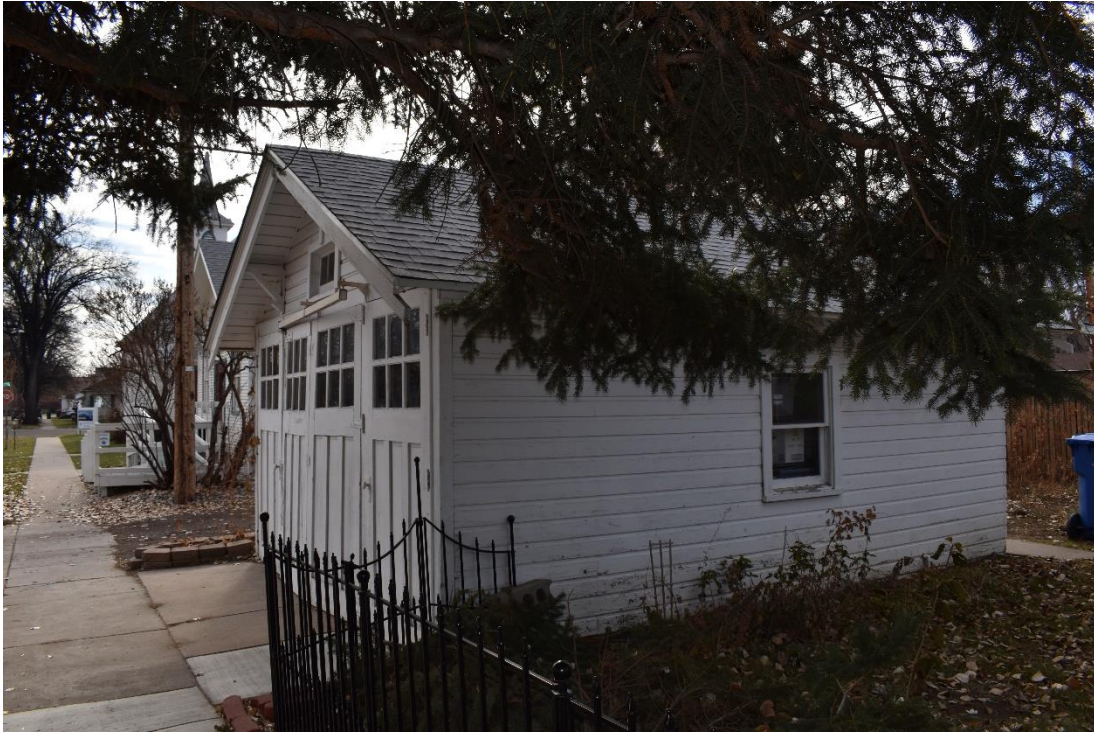
CD 1, Image 107, View to South-southwest, of the garage
