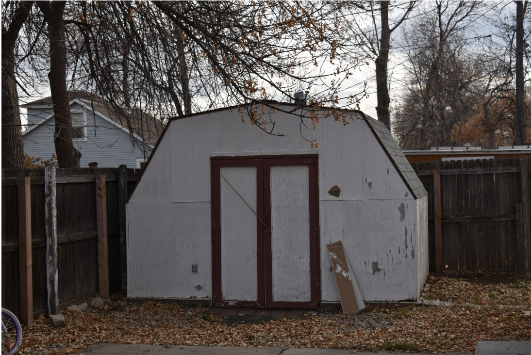
CD 1, Image 151, View to South, of the shed
