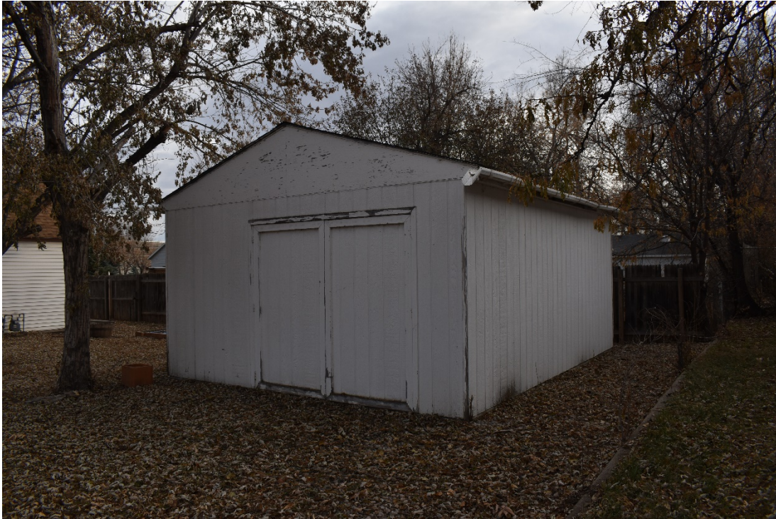
CD 1, Image 149, View to Southeast, of the garage
