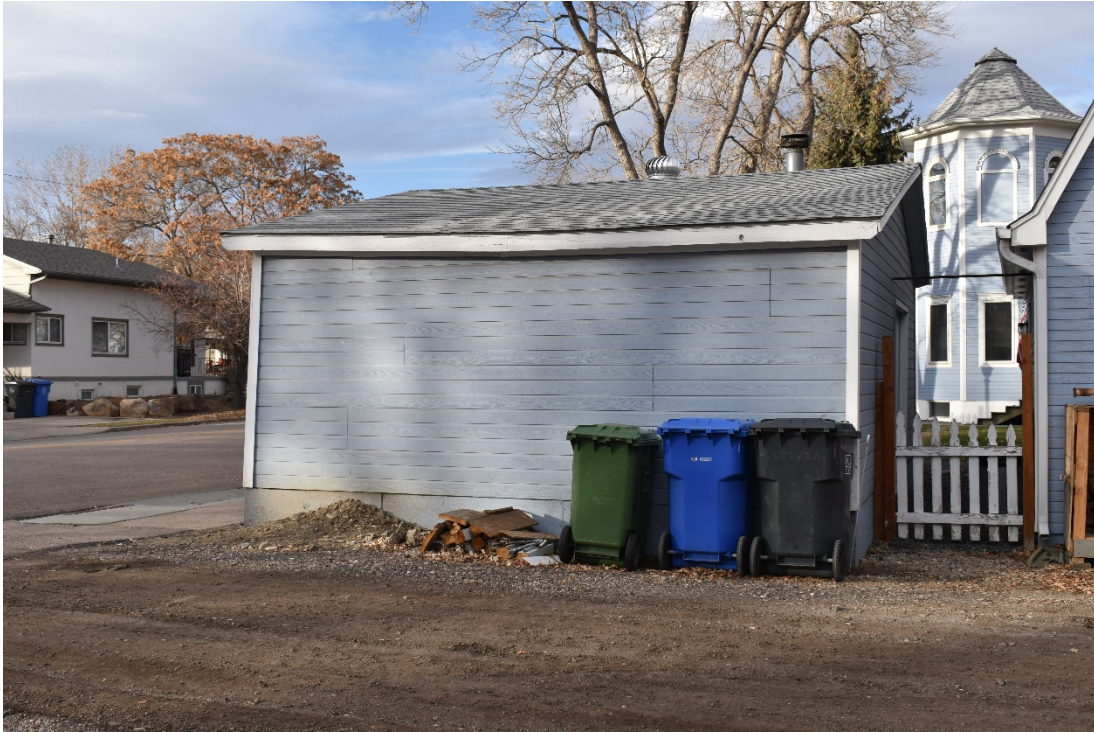
CD 1, Image 143, View to North, primarily of the gable-roofed garage
