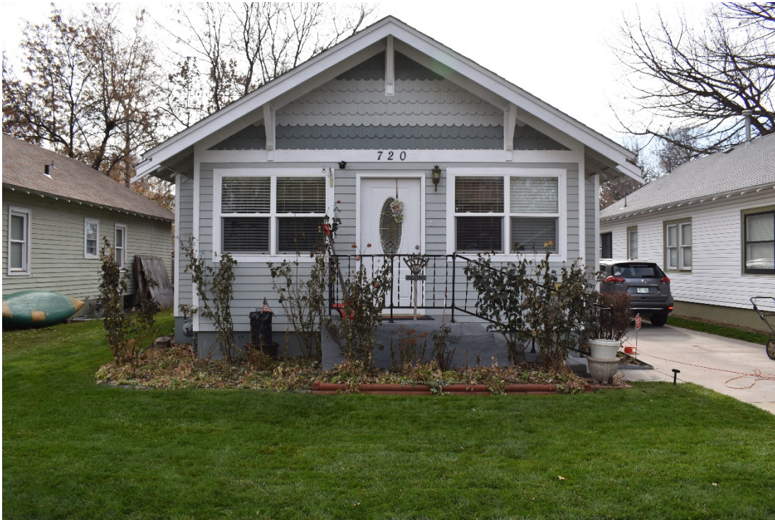
CD 1, Image 75, View to South, of the dwelling
