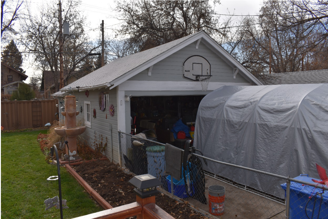
CD 1, Image 79, View to Southwest, of the garage
