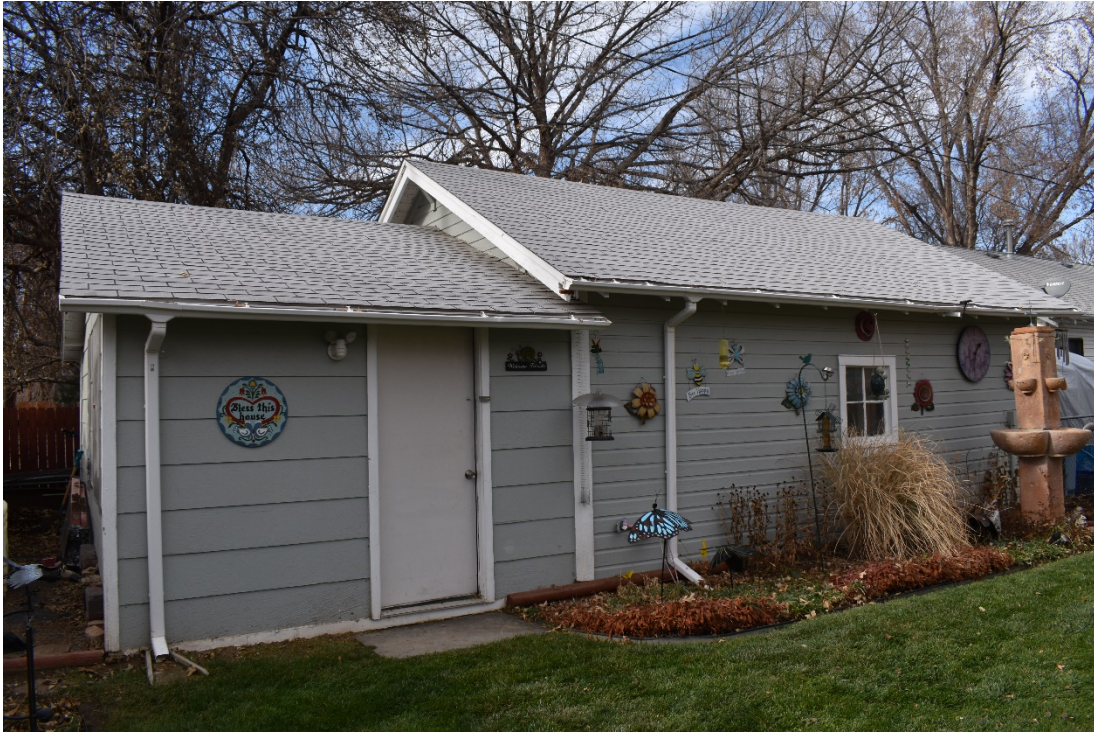
CD 1, Image 1, View to Northwest, of the garage
