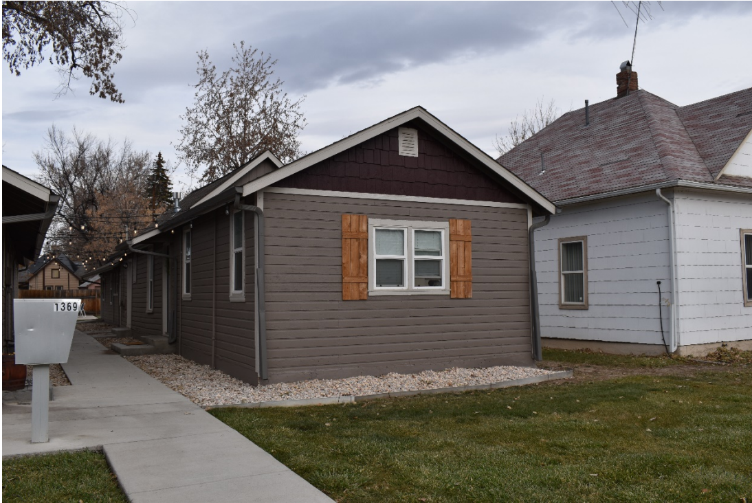
CD 1, Image 39, View to Northeast, primarily of the south and west walls of the east building
