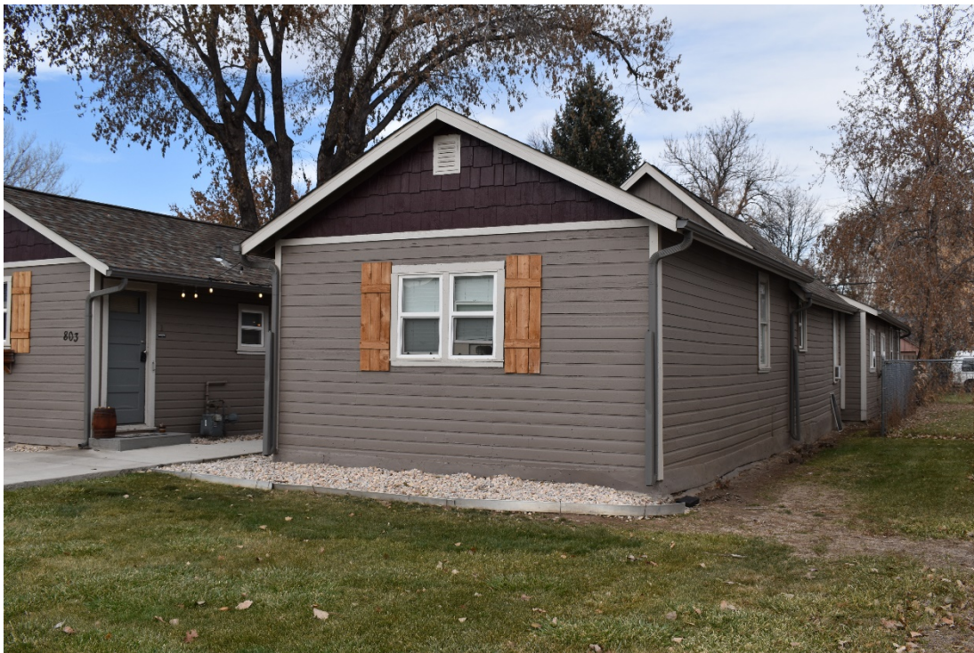
CD 1, Image 38, View to Northwest, primarily of the south and east walls of the east building
