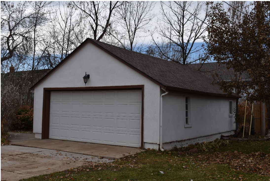
CD 1, Image 20, View to Southwest, of the Garage
