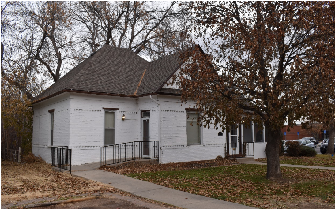
CD 1, Image 16, View to Northeast
