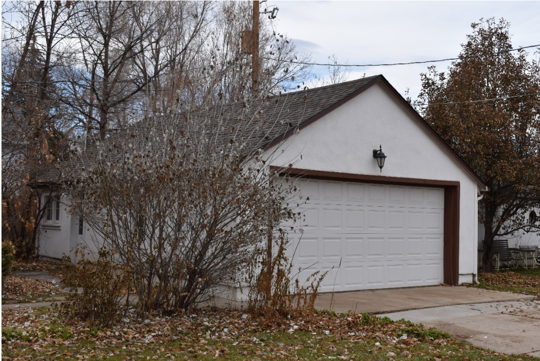
CD 1, Image 19, View to Northwest, of the Garage
