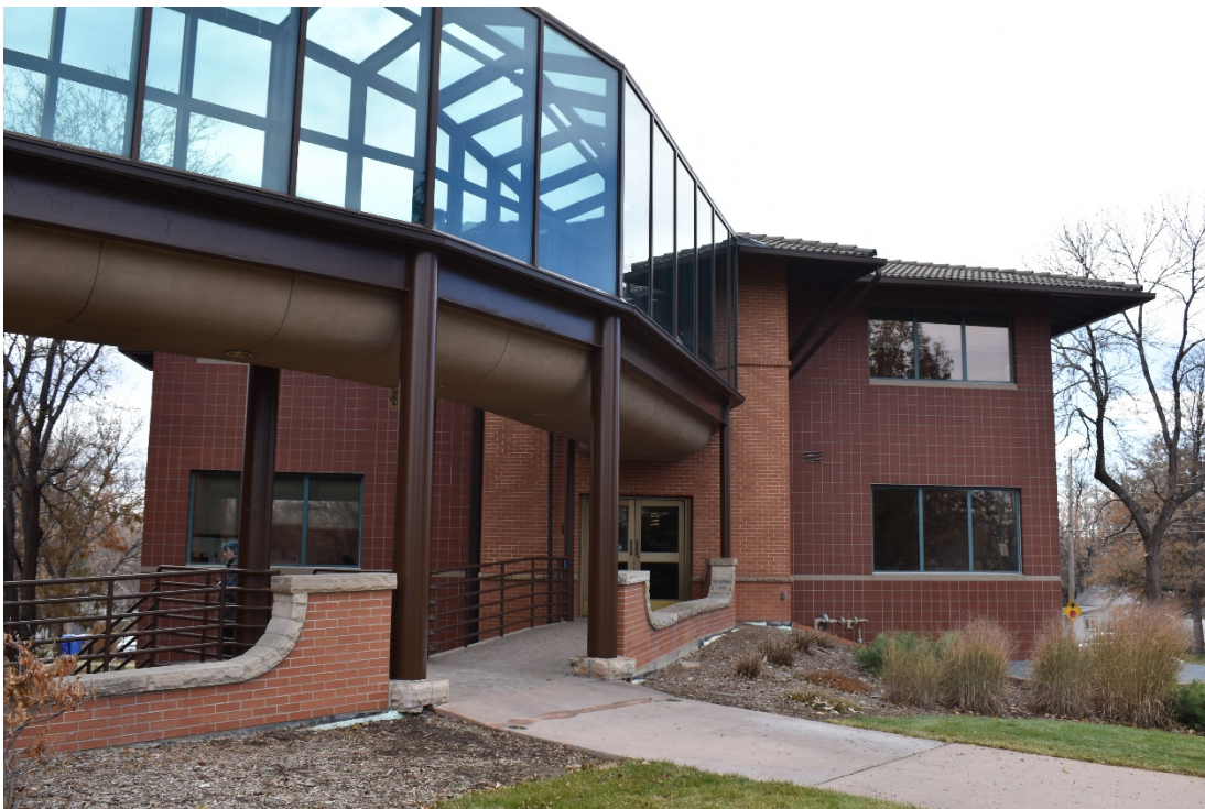
CD 1, Image 32, View to South, of the north wall of the Municipal Annex and of the walkway area
