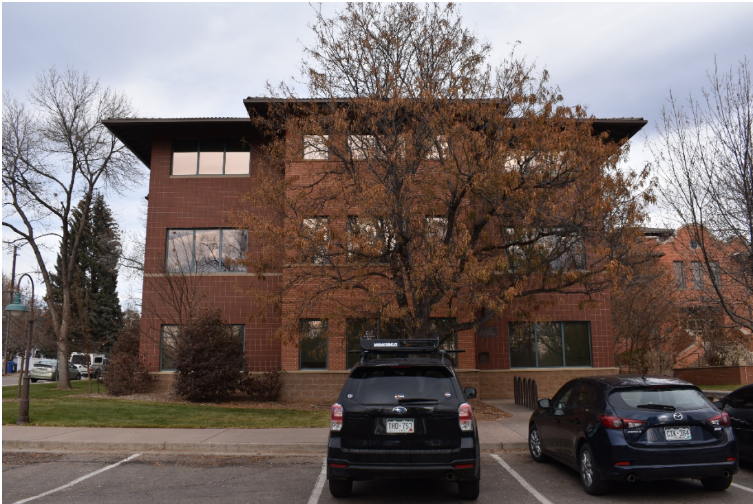
CD 1, Image 34, View to North, primarily of the south wall of the Municipal Annex
