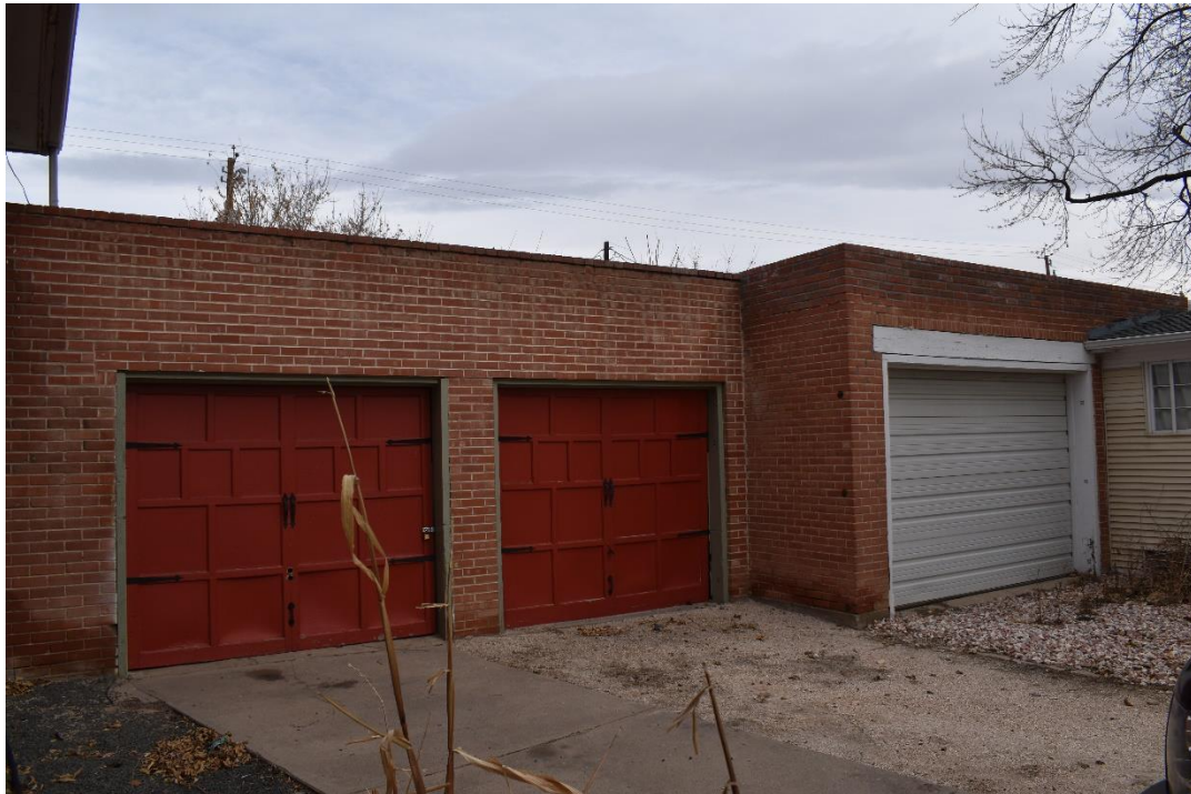
CD 1, Image 6, View to Northeast
