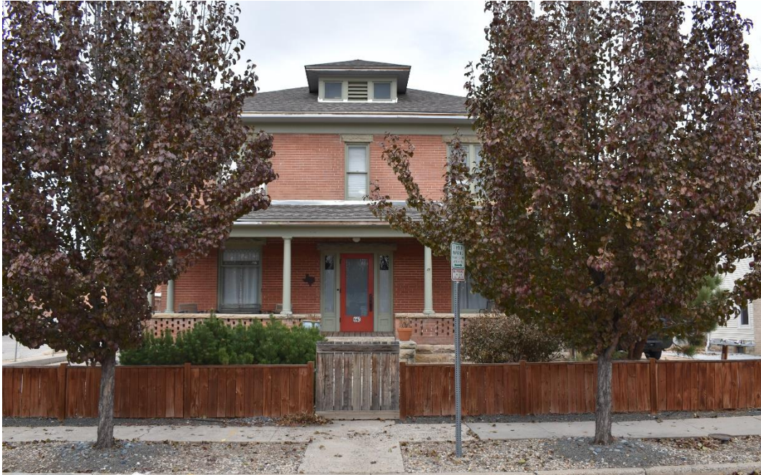
CD 1, Image 1, View to North
