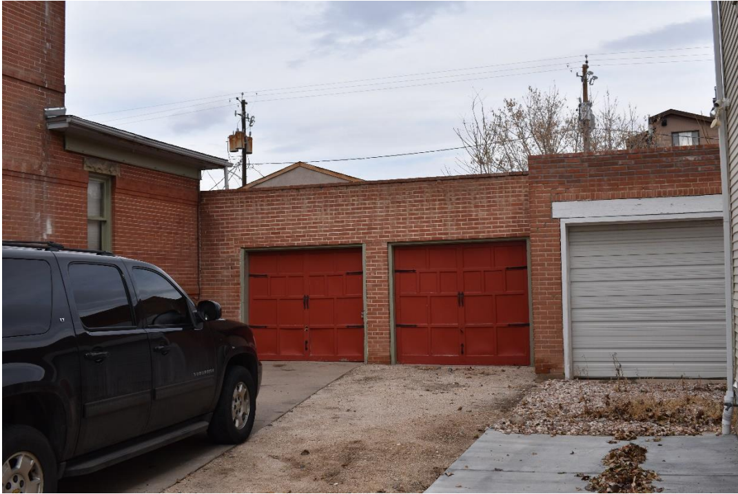
CD 1, Image 5, View to North
