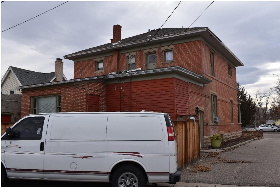
CD 1, Image 4, View to Southeast
