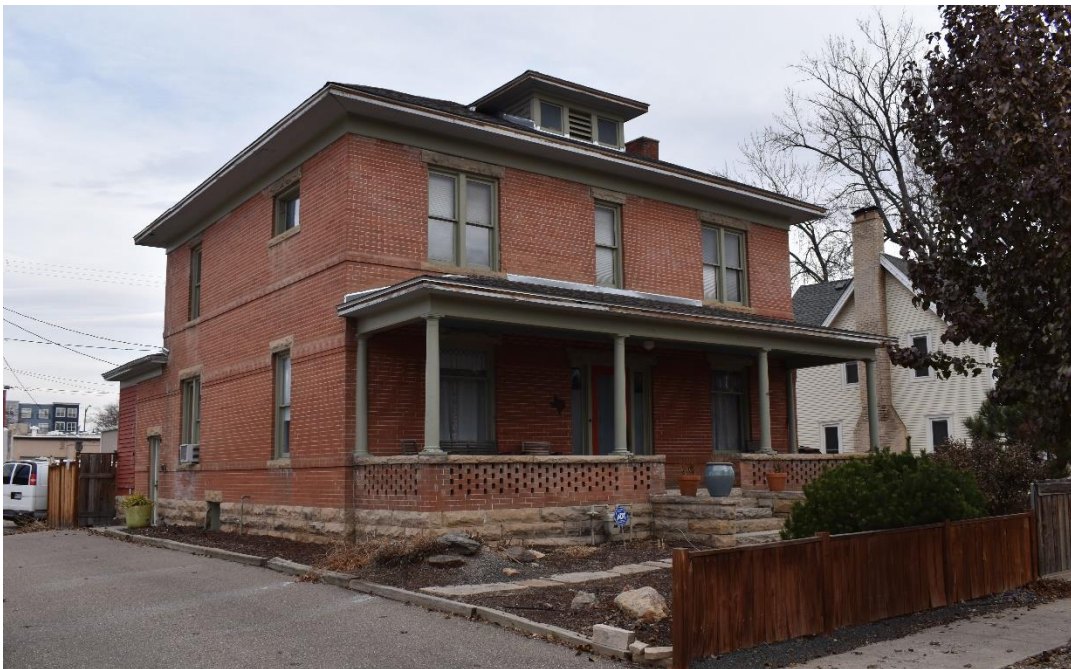
CD 1, Image 2, View to Northeast
