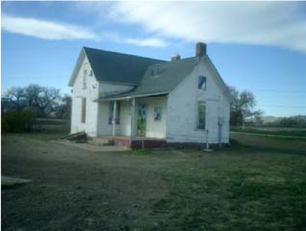
Fig. 10 2009 Northeast-facing side, prior to restoration
