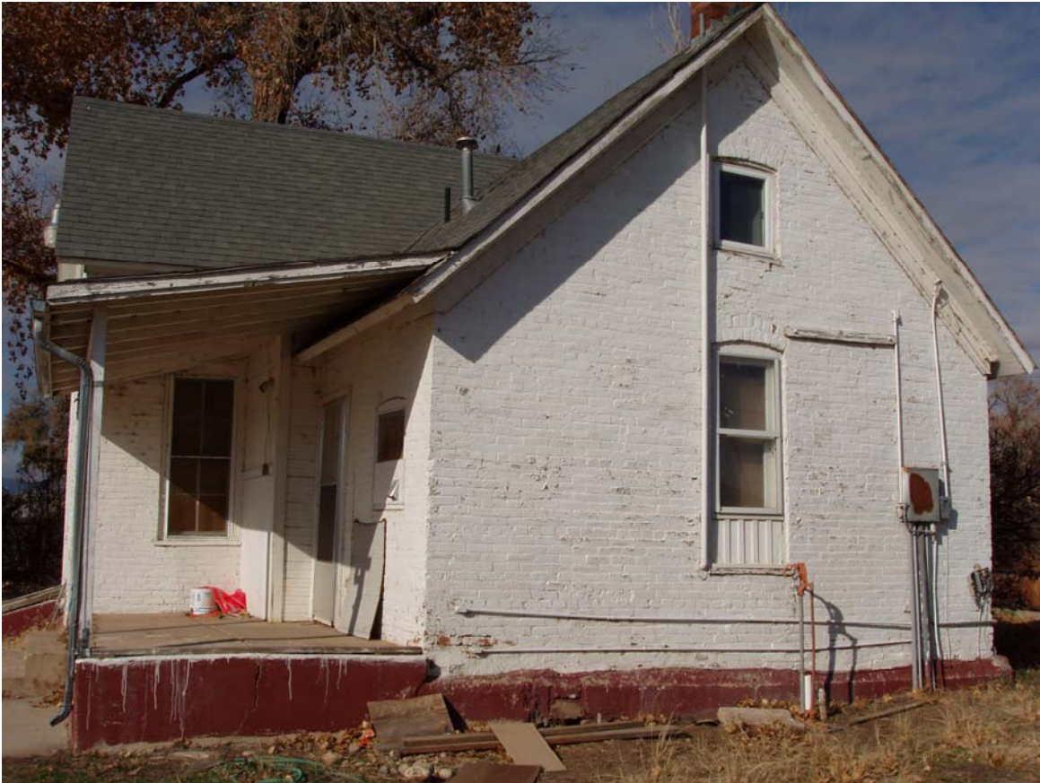
Fig. 8 2009 Northeast Façade, prior to restoration
