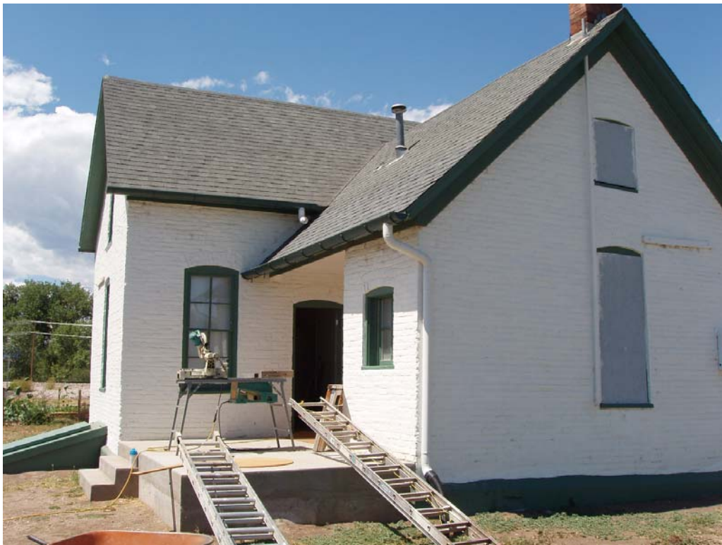
Fig. 19 2011 Northwest -facing side, during restoration
