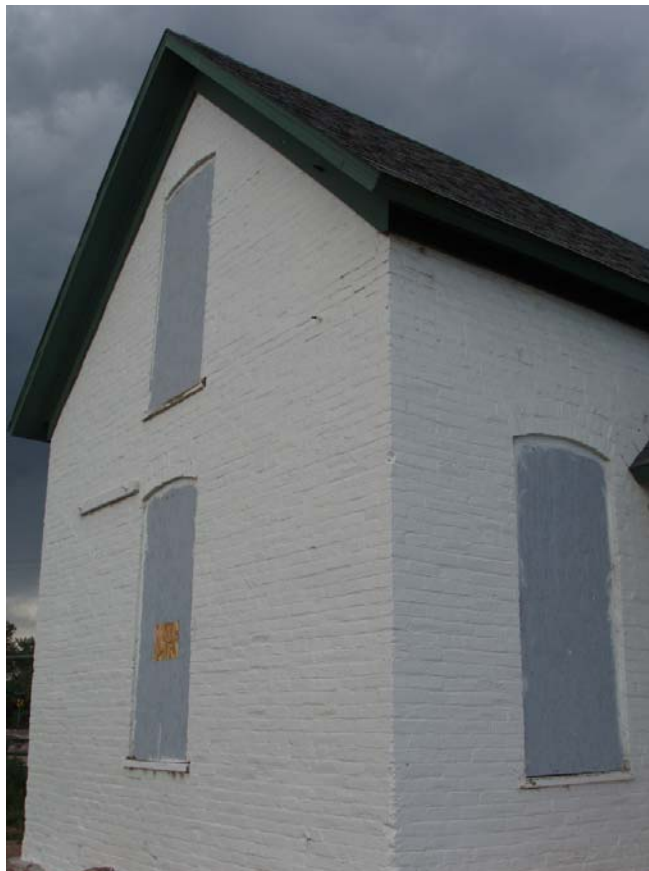
Fig. 13 2011 Southeast-facing side, during restoration
