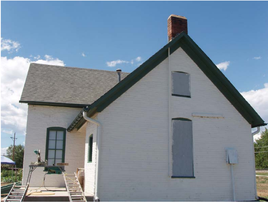
Fig. 18 2011 Northwest -facing side, during restoration
