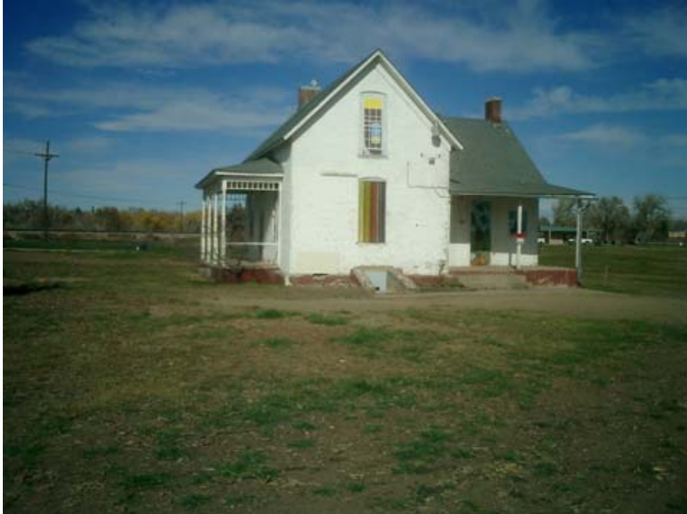
Fig7. 2009 Southeast -facing side, prior to restoration
