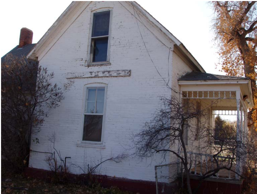
Fig. 6 2009 Southwest (main) Façade, prior to restoration
