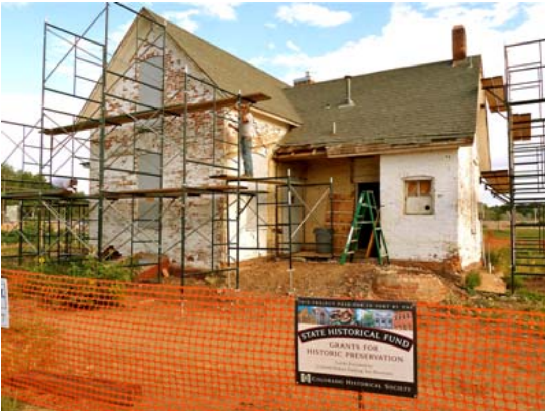
Fig. 11 2010 Southeast Façade, during restoration
