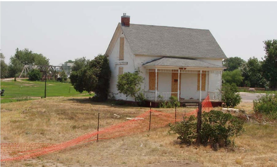
Fig. 9 2009 Southwest (main) Façade, prior to restoration
