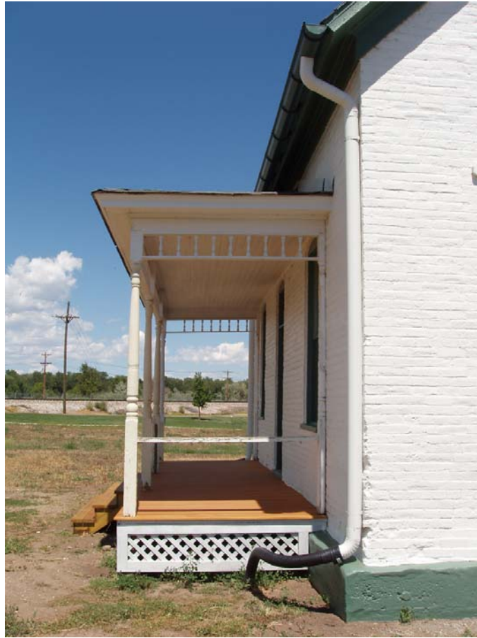
Fig. 16 2011 Southwest Porch, during restoration
