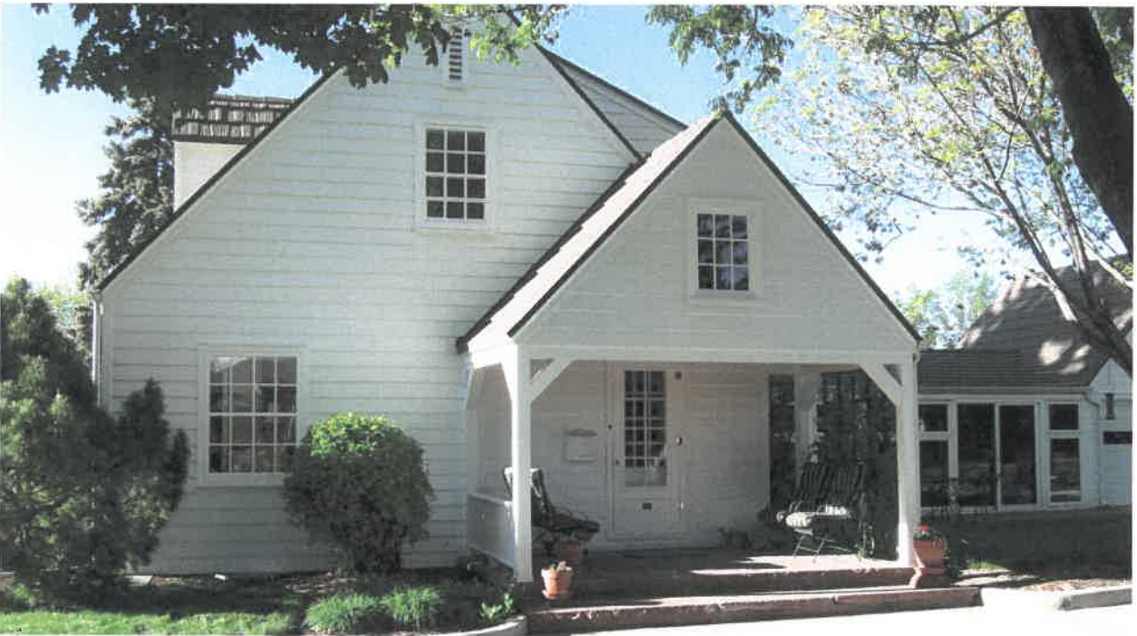
Photo 6: South side of house. June 2019.
