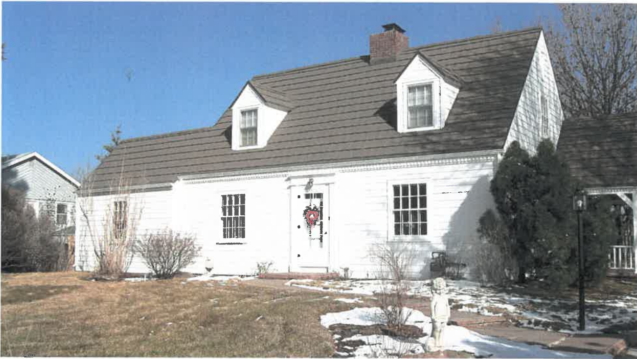
Photo 2: West (front) side, 1953 north addition at left. February 2019.
