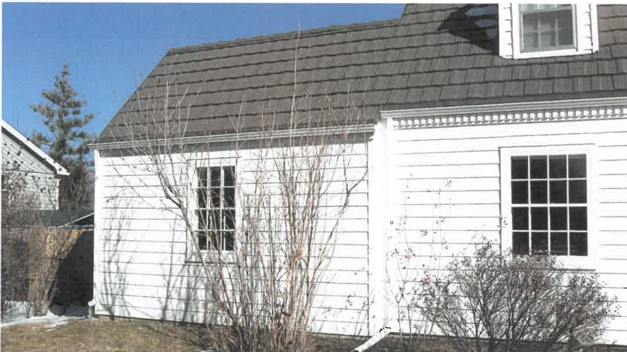
Photo 4: West (front) side of 1953 north addition. February 2019.
