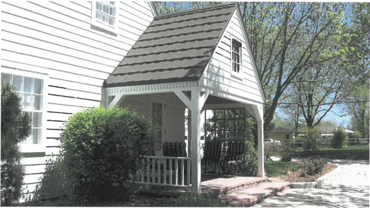
Photo 5: South porch with dentil work at roofline and “ghost room” above. August 2017.
