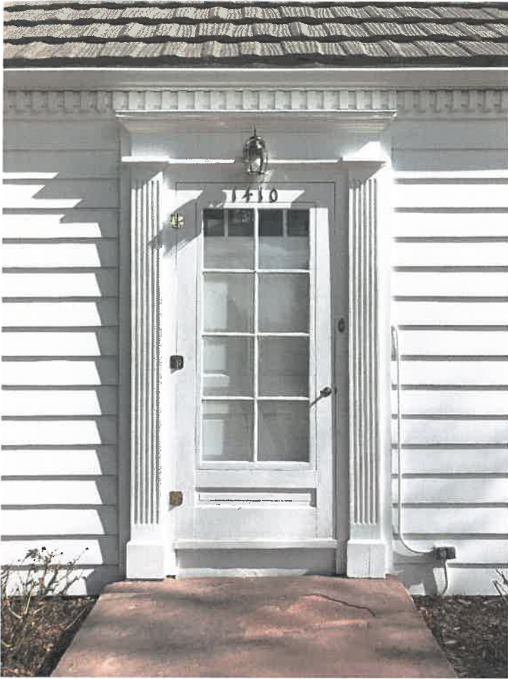
Photo 3: Entry with historic storm door and classical door surround. Note dentil details at roofline. Photo by Amy Unger, February 2019.
