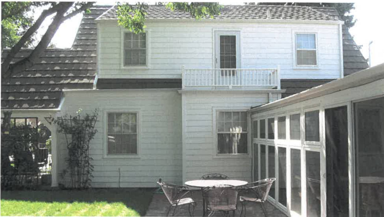
Photo 8: East side of the house. Note balconette at second floor. August 2017.
