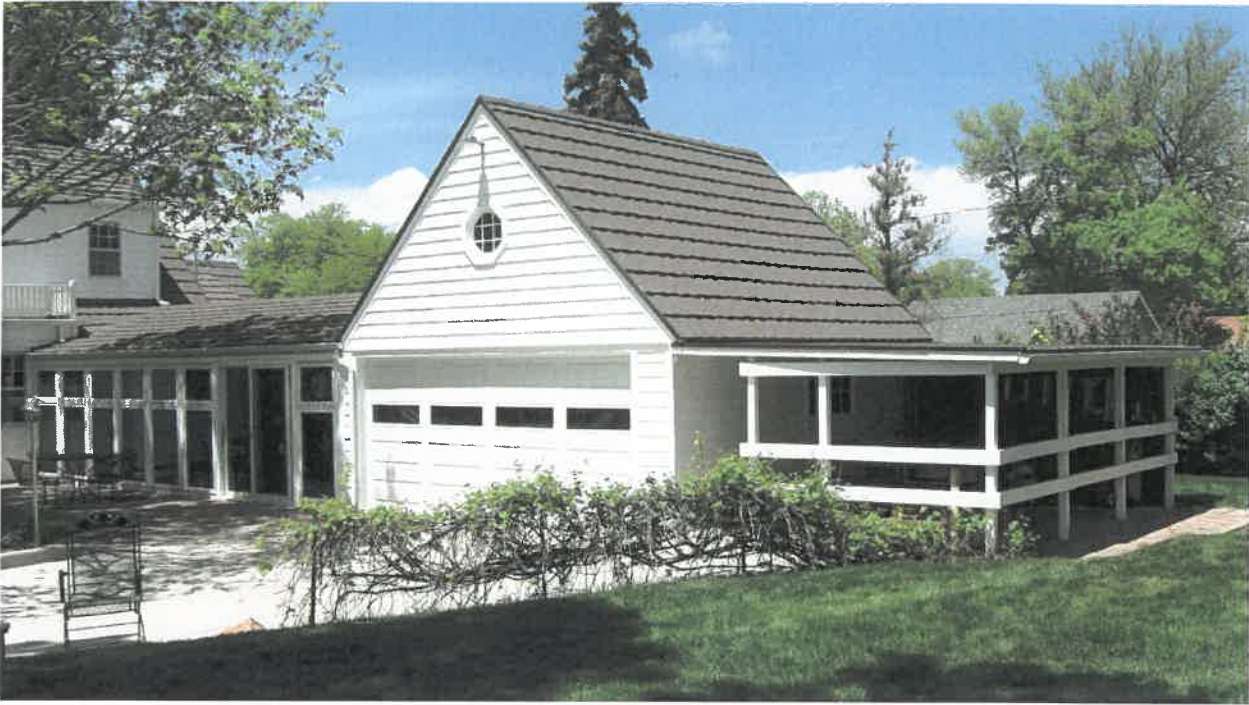
Photo 9: South side of enclosed breezeway, garage with octagon window at gable end, and attached covered storage area. June 2019.
