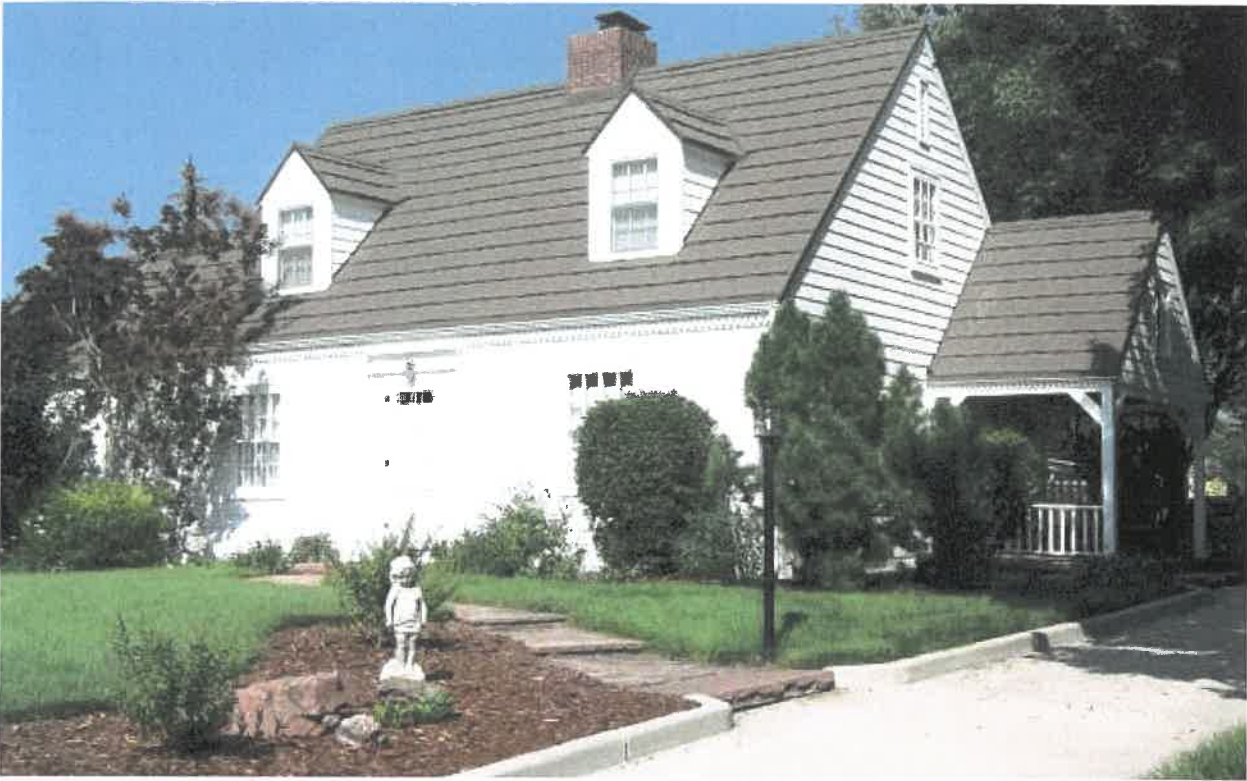
Photo 1: West (front) side, south porch at right. August 2017.
