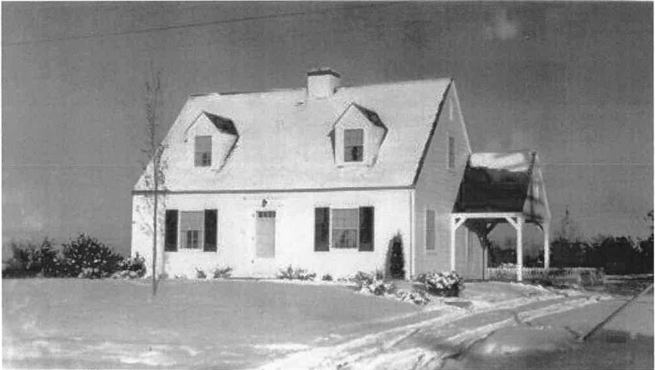
Figure 1: The Kelley House, winter, 1940. (Photograph courtesy of Betsy Anne Kelley)
