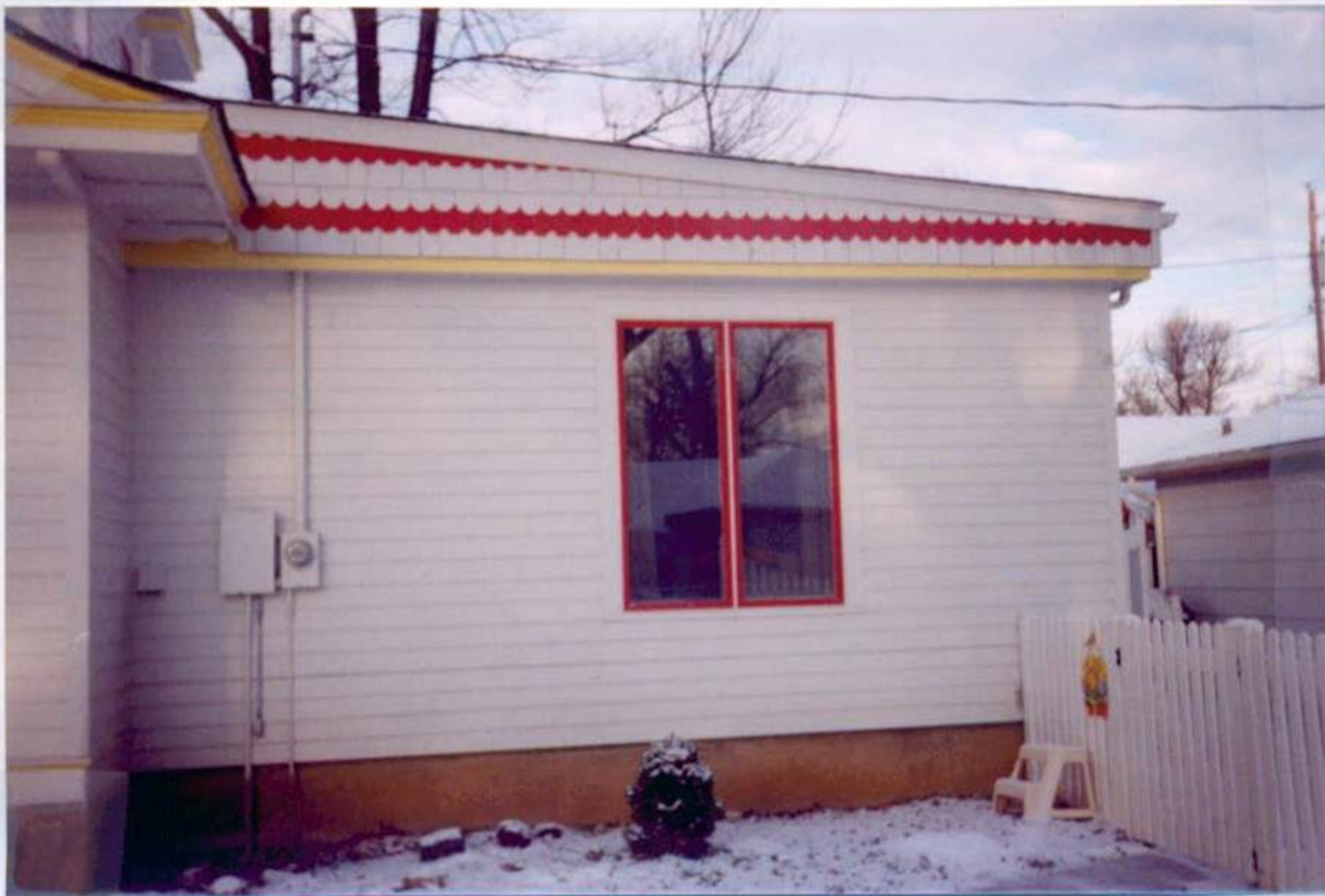
Family Room addition
