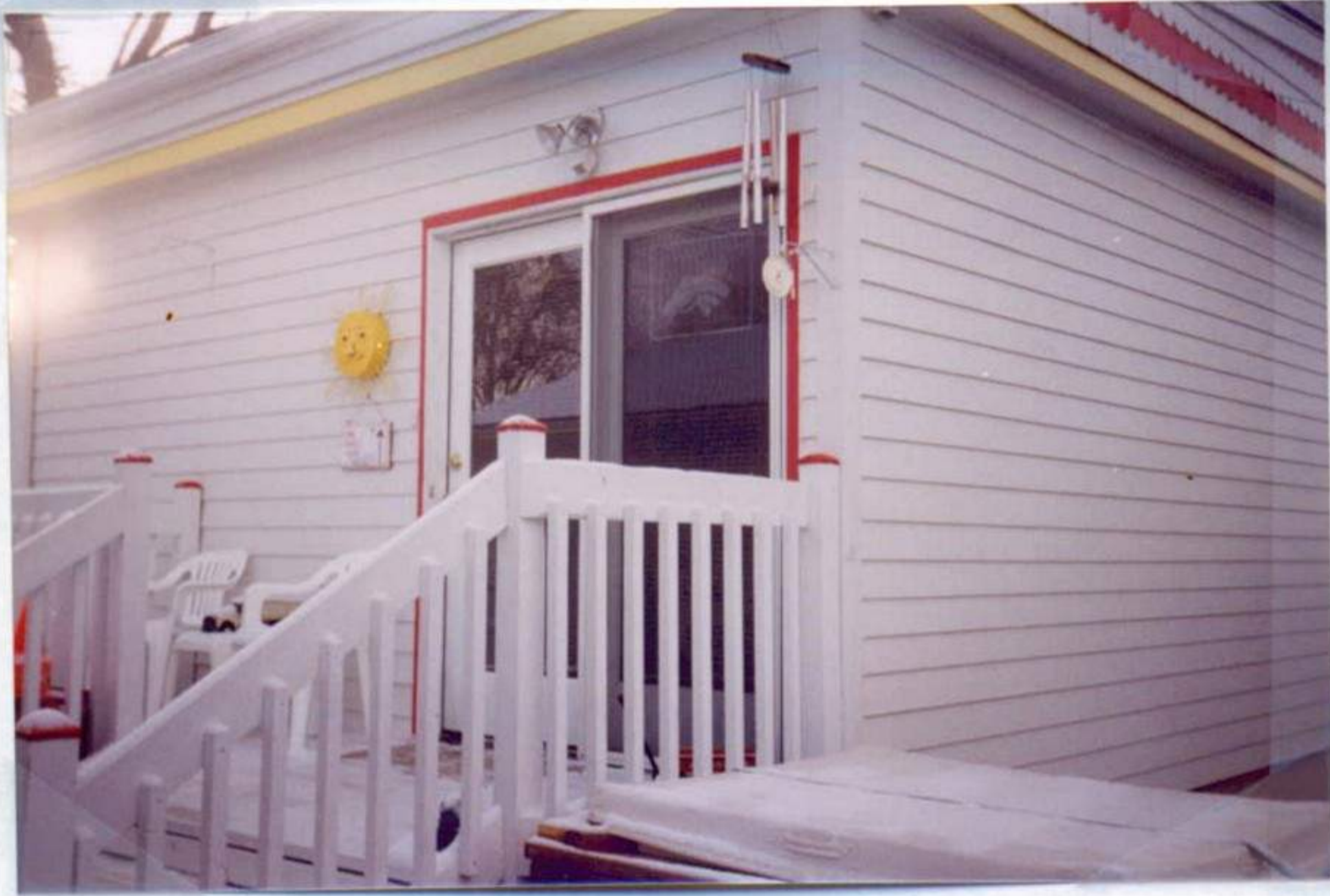
Back Deck addition
