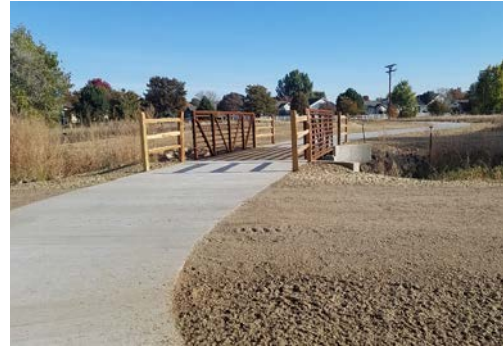
New Madison Avenue bridge and trail
