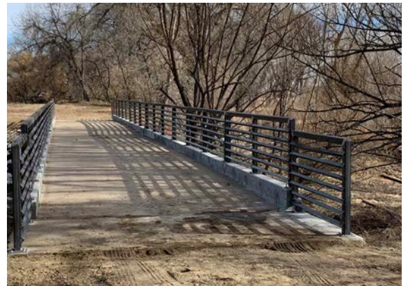
Refurbished pedestrian bridge at Oxbow Natural Area
