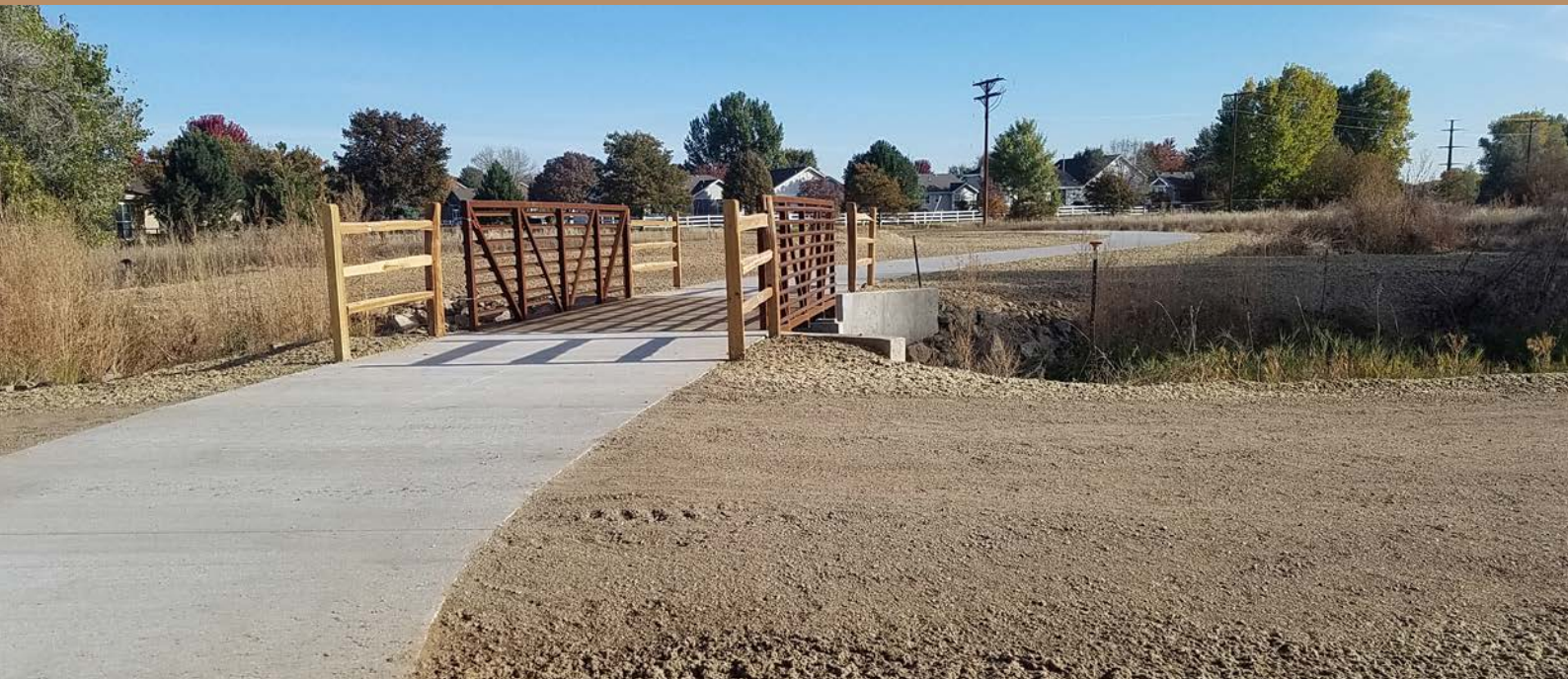
New Madison Avenue bridge and trail connection to Old St. Louis
