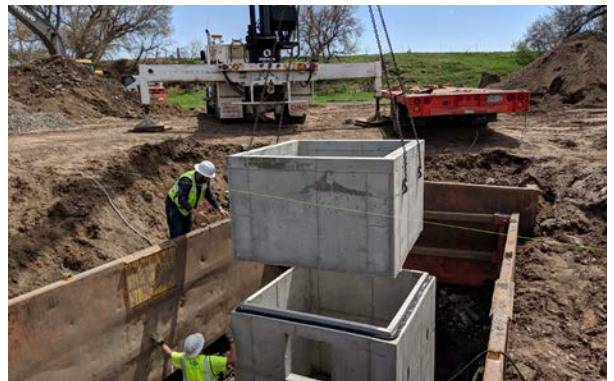
Wet well installation for new Medina's Crossing pump
