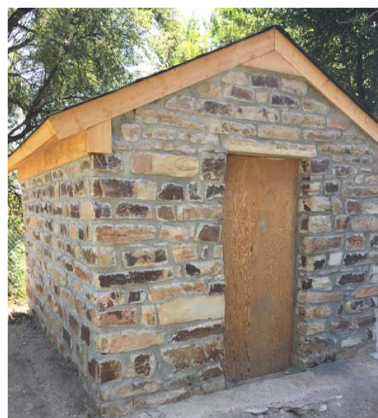
Restored historic structure at Sunset Vista Natural Area
