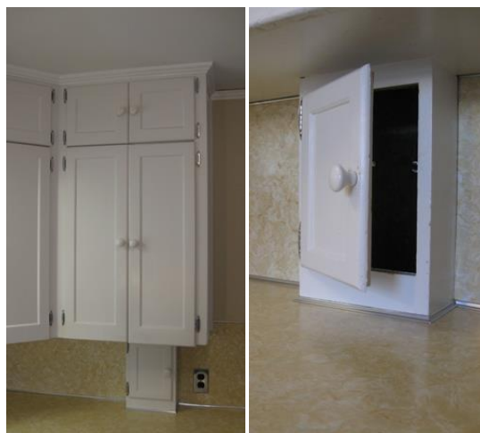
3-29. Laundry chute access in the kitchen.
