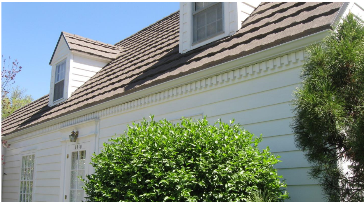
3-2. Architectural dentil work on the front of the house.
