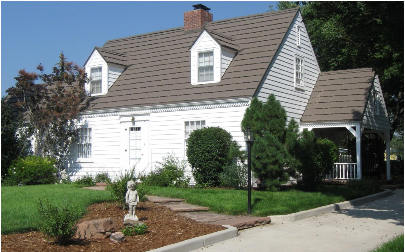
3-1. Exterior of the Cape Cod style Kelley-Coffman House at 1410 North Garfield Avenue.
