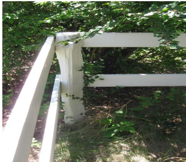
3-8. Example of hand hewn wooden fence posts supporting the fence on the east and the south property boundaries.
