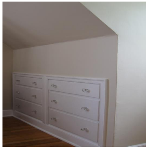
3-30. Built-in drawers in both second floor bedrooms use space beneath the steep sloping roof.
