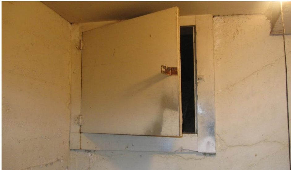
3-33. Root cellar in the basement.
