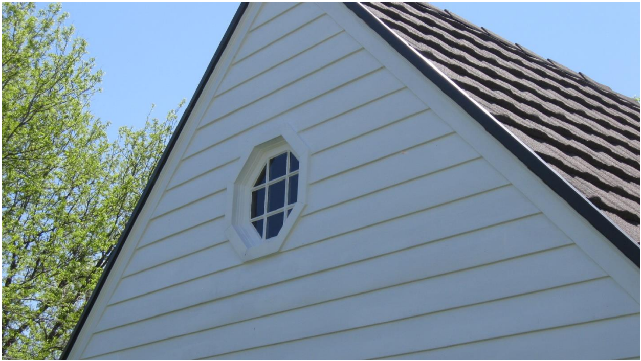
3-7. Octagonal window on the north side of the carriage house.
