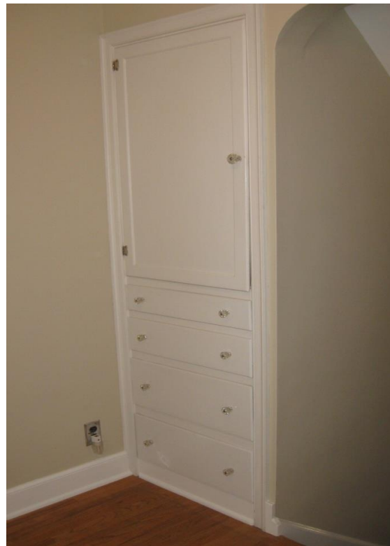
3-31. Built-in drawers and cabinet on the second floor landing.
