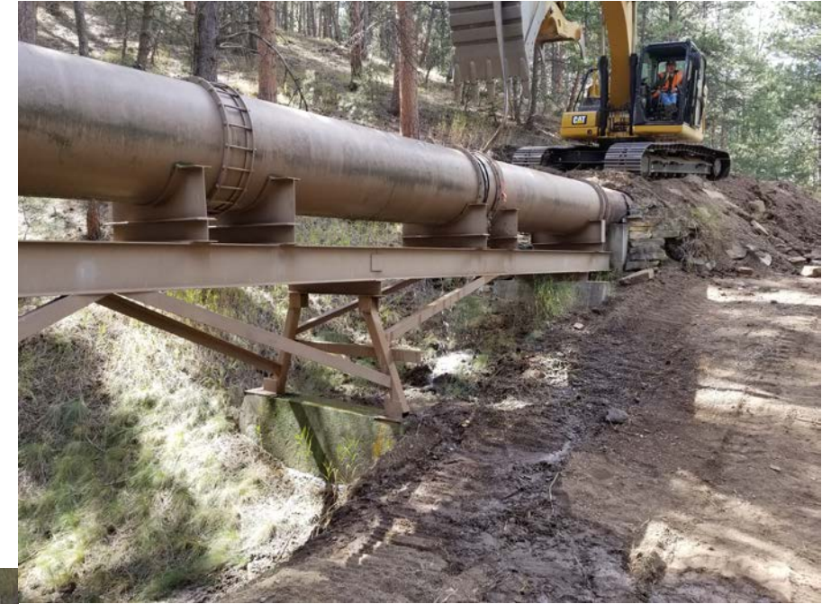
Trestle and Pipe Dangling by the Ends
