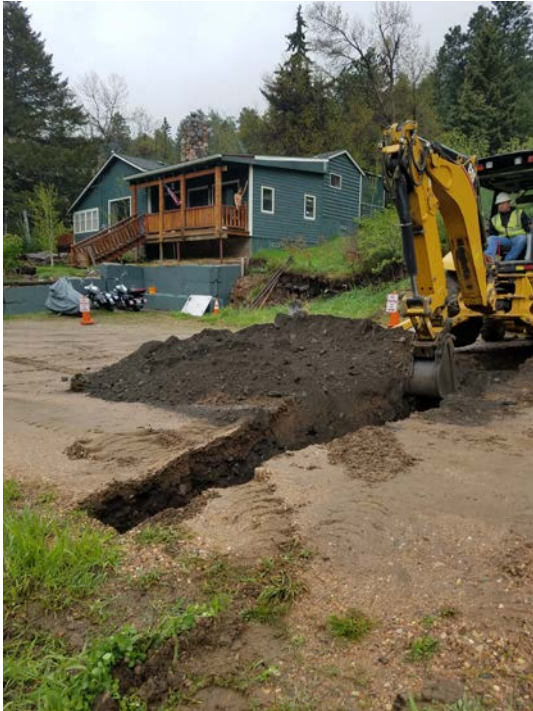
Dragging for pipe
