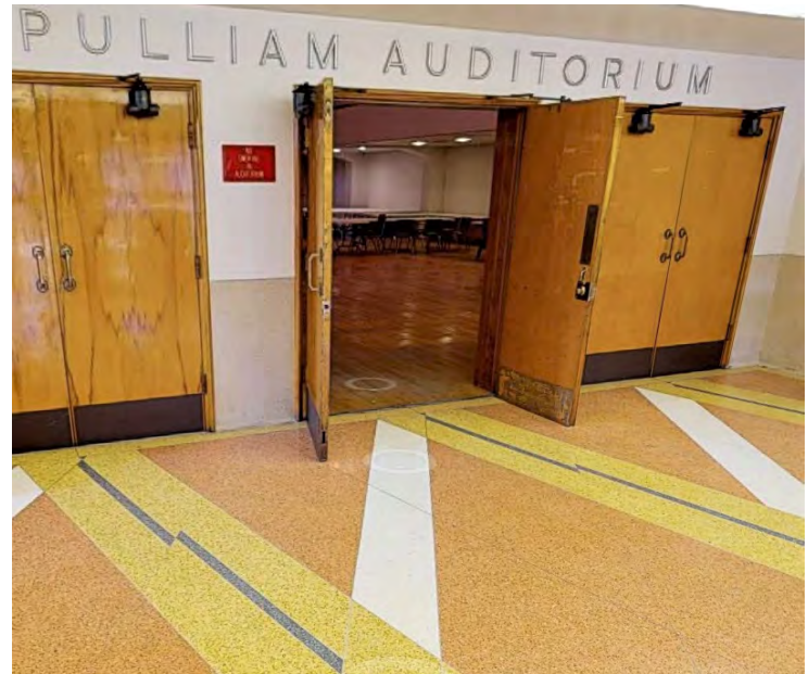
The original Terrazzo flooring in the upper and lower lobbies of the Community Building will be restored, repaired and polished during the second phase of construction on the building.
