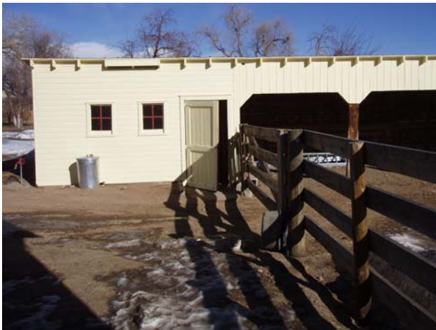
South Elevation (west side)
