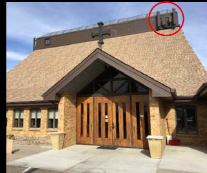
Small Cell Wireless Facility on private property
