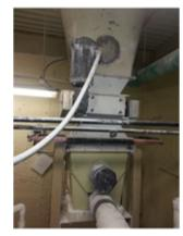
With the recent Water Treatment Plant expansion project a new chemical building and chemical feed system was put into operation. Soda ash is used to adjust the pH of the water. The no longer used old soda ash storage and feed area needs to be rehabilitated to meet the current needs of the facility.
