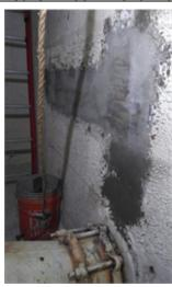
Water Treatment Plant Filter Building 2 Concrete Wall Repair Filter Building 2 at the Water Treatment Plant (WTP) provides half of the filtering capacity for the City of Loveland. The concrete housing the filters has aged and portions have become soft, degraded, and there have been isolated leaks. Repair of the aging and failing portions of the concrete will be repaired.
