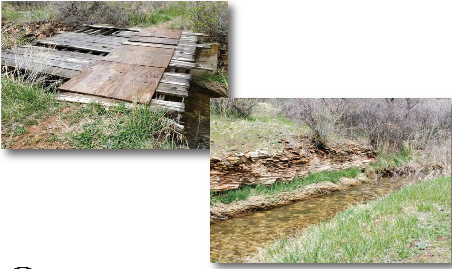
① Existing Louden Ditch crossing
