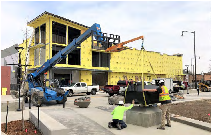
A black granite shell, covering the concrete base for a clock tower donated by the Loveland Rotary Club, is lowered into place. The MetroLux Dine-In theater is under construction in the background.
