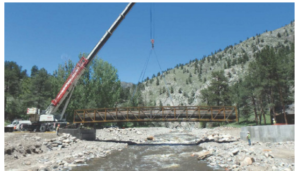
Placement of a new 100-foot-long pedestrian bridge
