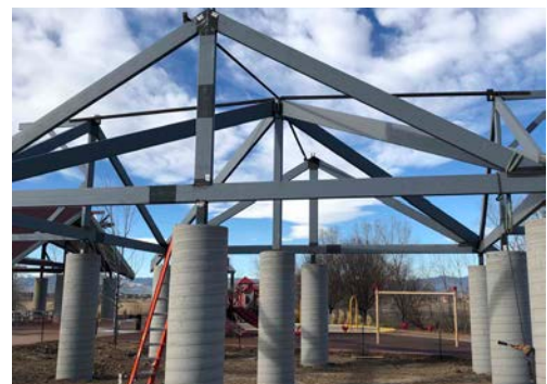
LSP Phase II construction
