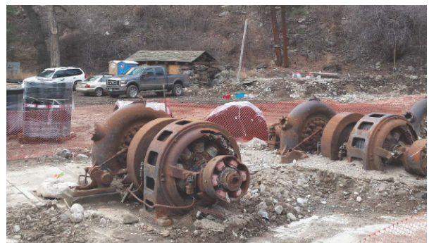
Historic power generators
