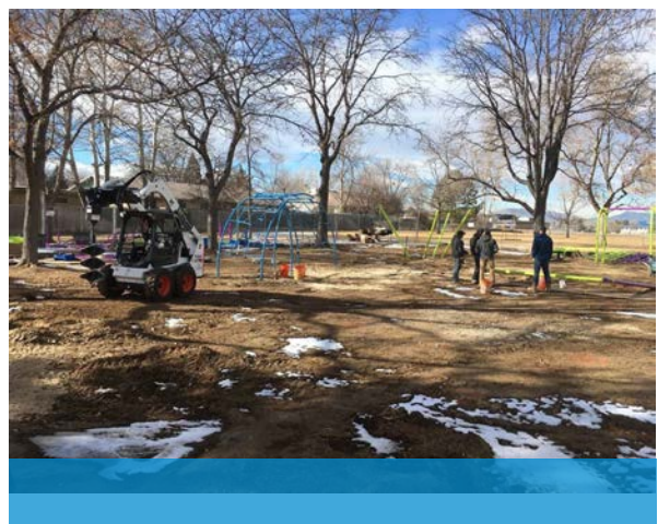
New ADA-accessible structures being placed at Silver Glen Park
