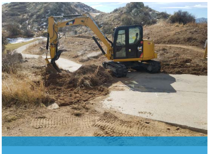
Excavating for new cart turnarounds at Mariana Butte
