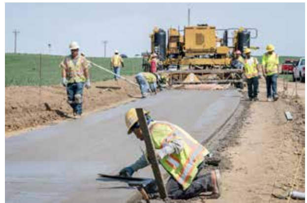
Long View Trail construction, photo by Rod Cerkoney
