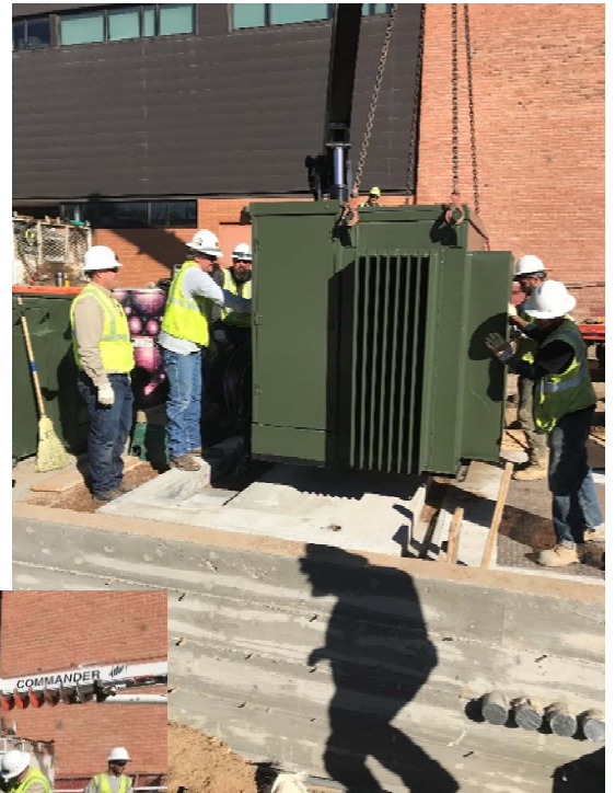
Secondary connection cabinet set on top of the new vault
