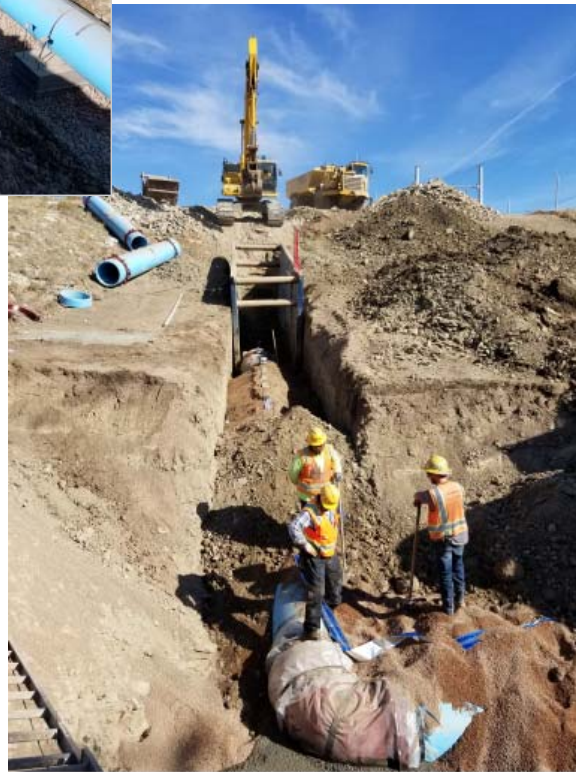
Water main being installed uphill toward the 29 th Street Tank
