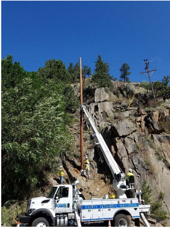
Power Contracting setting 55' pole for the 12.47 kV line crossing Hwy 34
