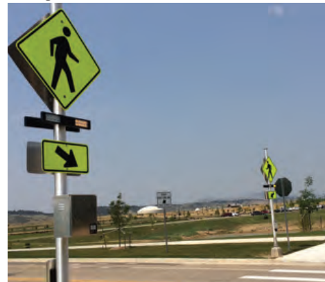
Flashing beacons at 22nd Street flash when pedestrians or cyclists push a button.
