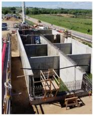
Other notable construction activities include the continued progress on the new return activated sludge (RAS) anoxic tank (pictured left). The tank structure is scheduled to be complete by late summer. The rehabilitation of the third secondary clarifier is nearing completion, which includes the sandblast and re-coating of the rotating mechanism as well as other performance enhancements.
