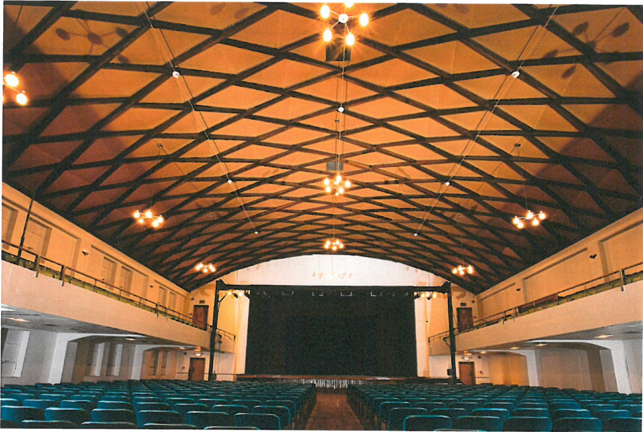
Figure 6. The Pulliam Auditorium with the Lamella Truss Roof
