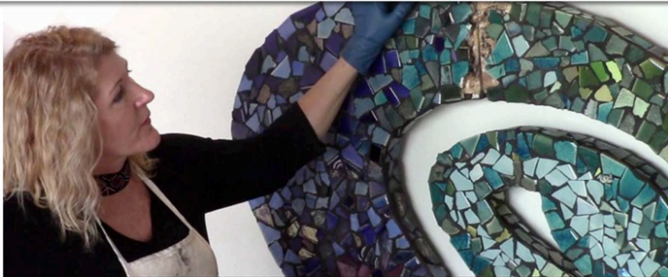
Annette Coleman reinstalls the work "Water Dreams" in the lobby of the Broomfield Health & Services building.
